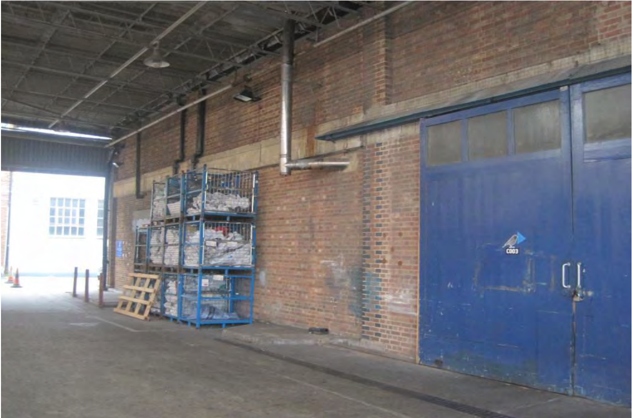
Photo No 23: Delivery bay entrance door to Building B
