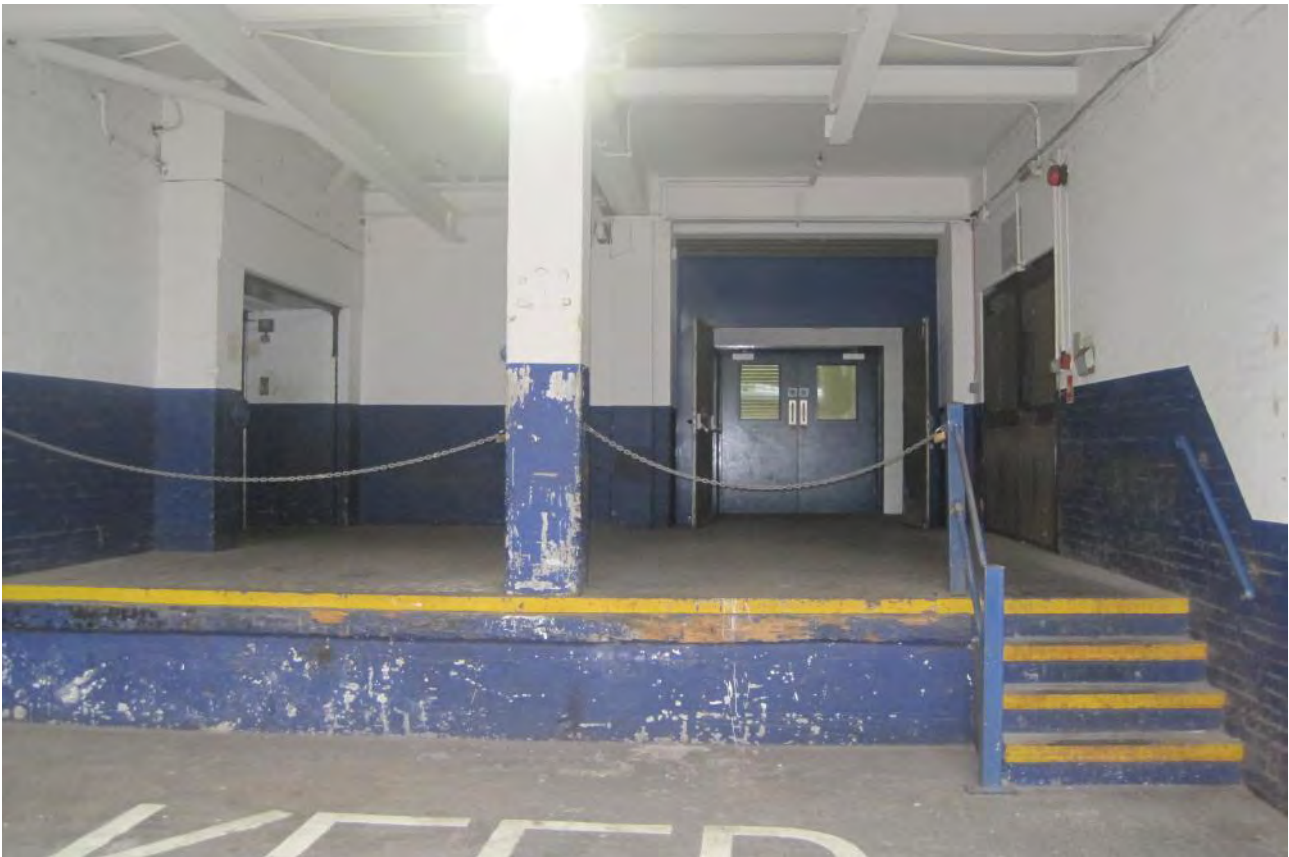
Photo No 9: Loading bay to side elevation of Building A
