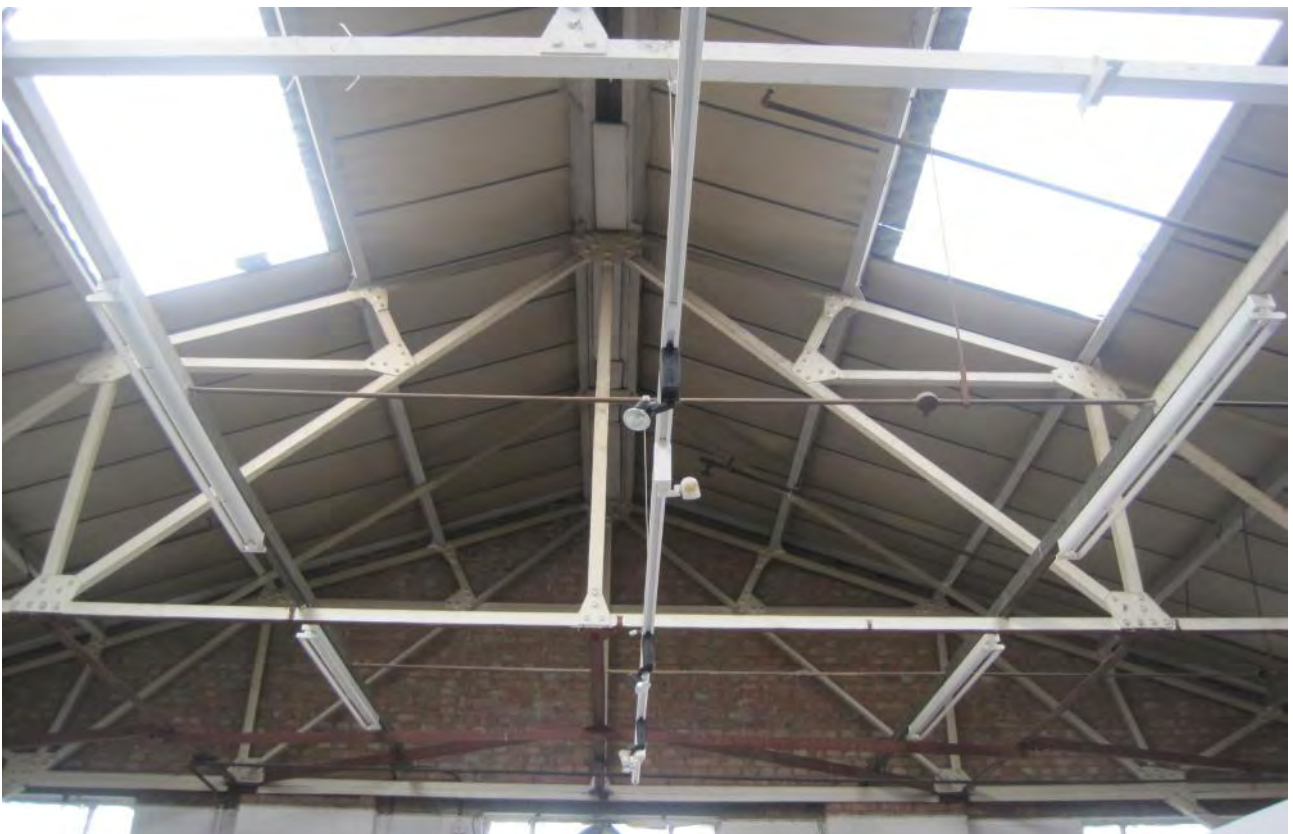
Photo No 24: Roof trusses and soffit lining panels to Building C
