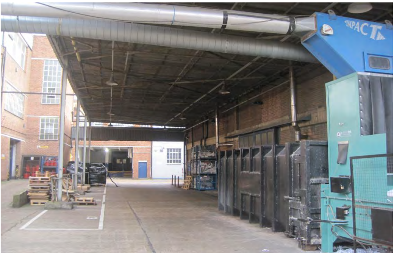
Photo No 22: Covered delivery bay area to Building B
