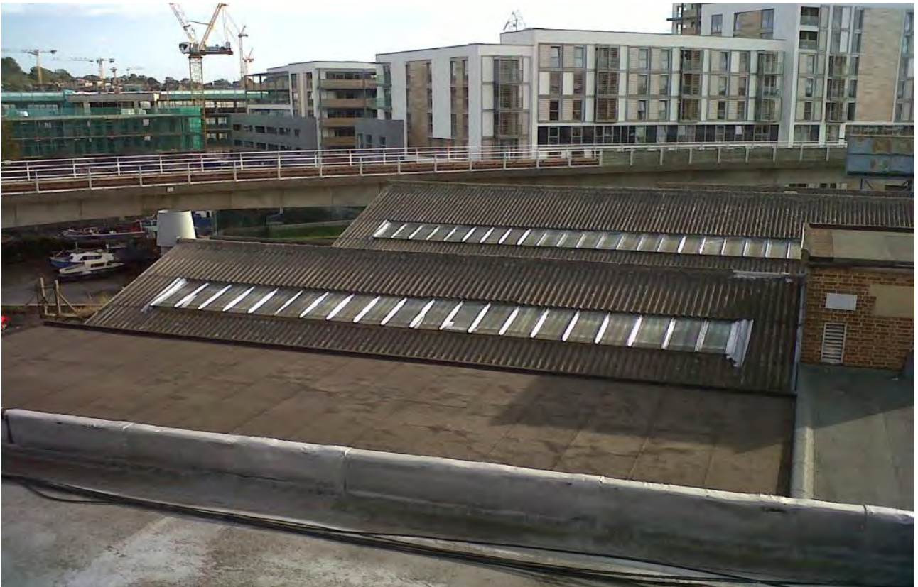
Photo No 2: Rear section of Building A
