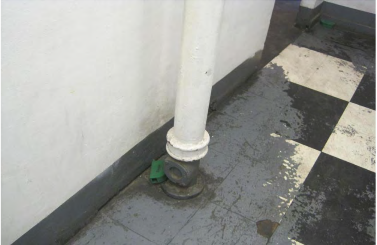
Photo No 17: Internal rainwater downpipe to Building B
