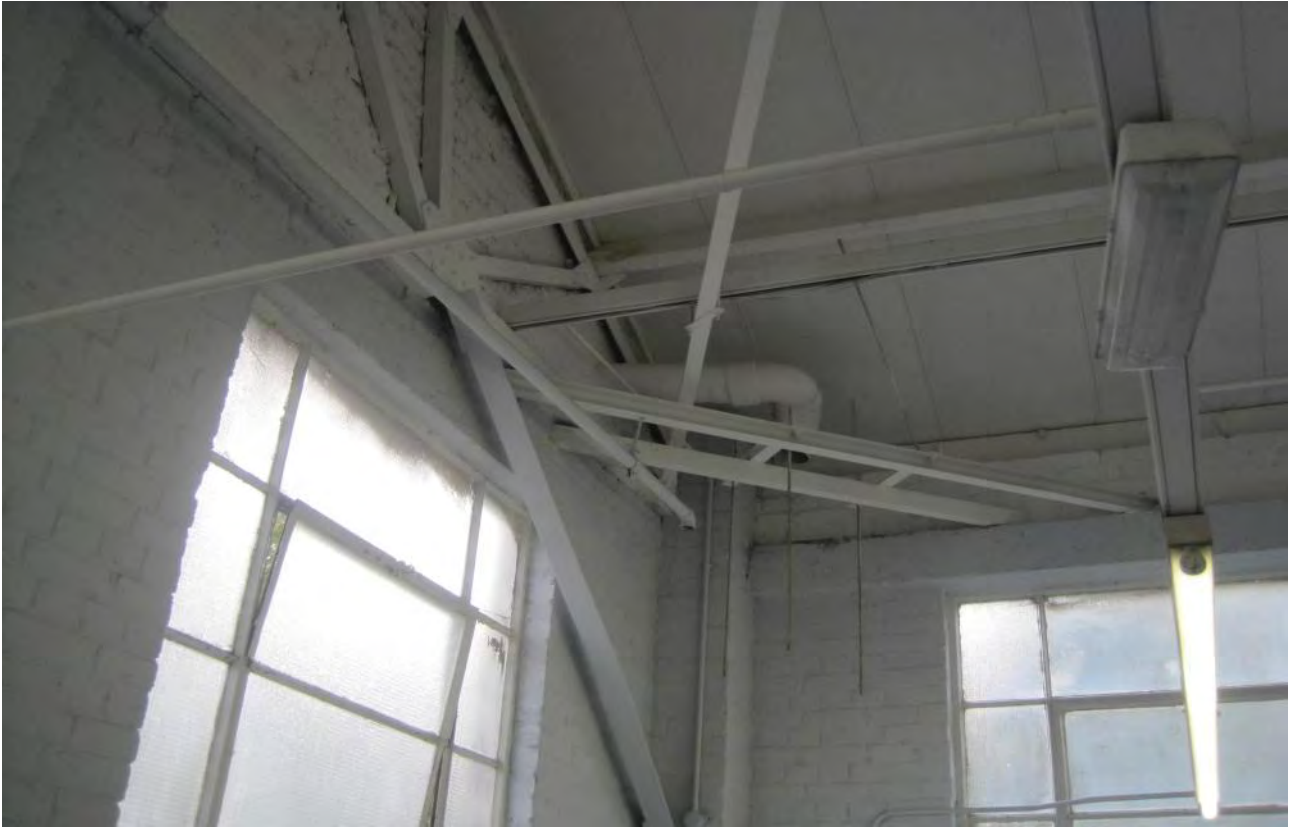
Photo No 25: Painted brickwork and steel trussed roof to Building C
