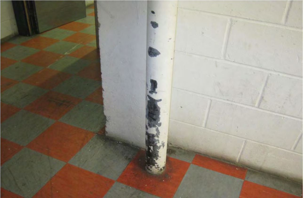
Photo No 13: Internal rainwater downpipe to Building A
