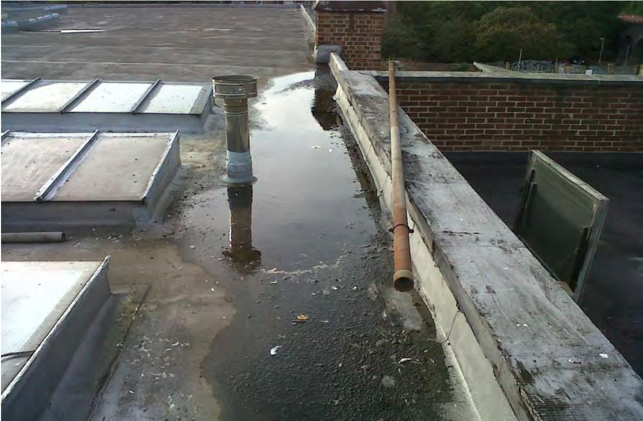
Photo No 3: Patch repairs to building B
