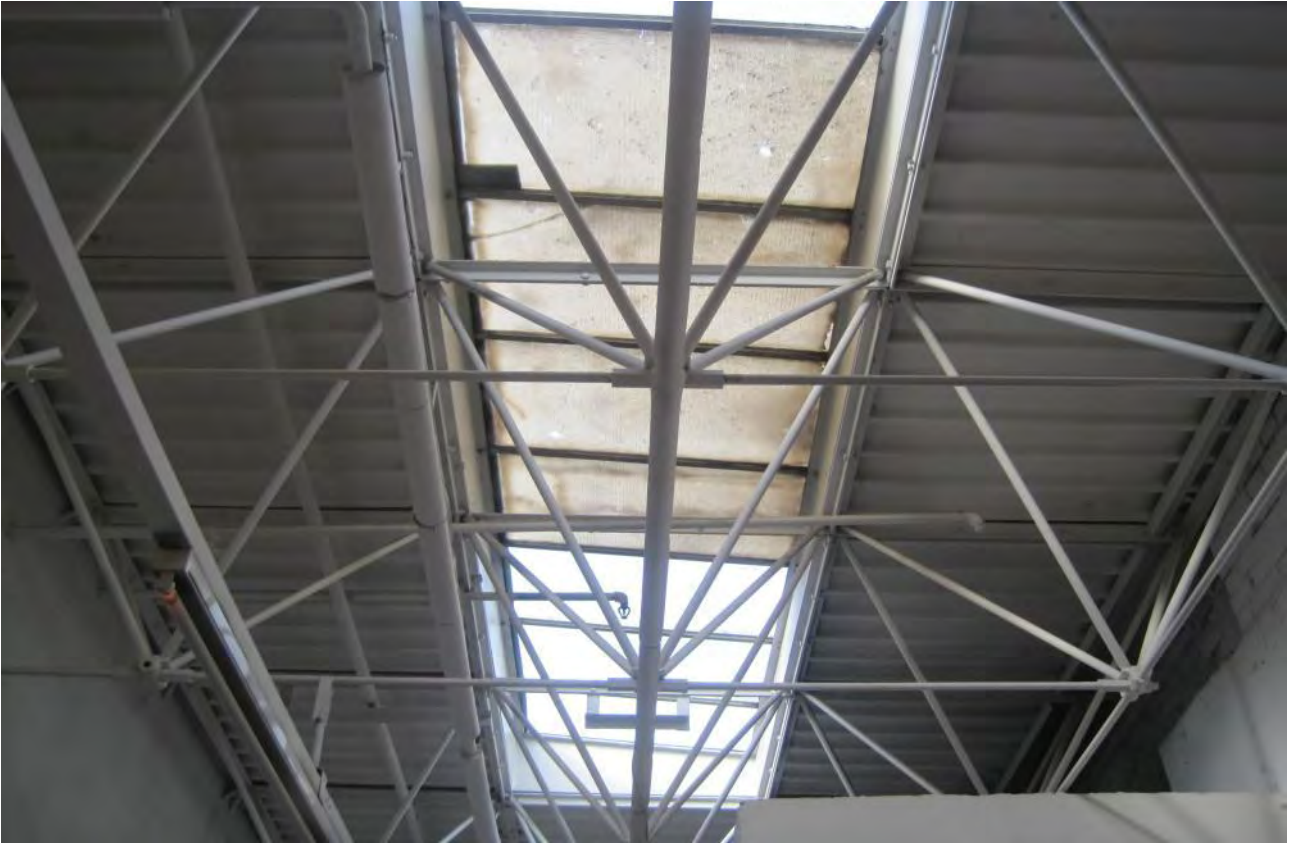
Photo No 19: Space frame roof trusses to building B
