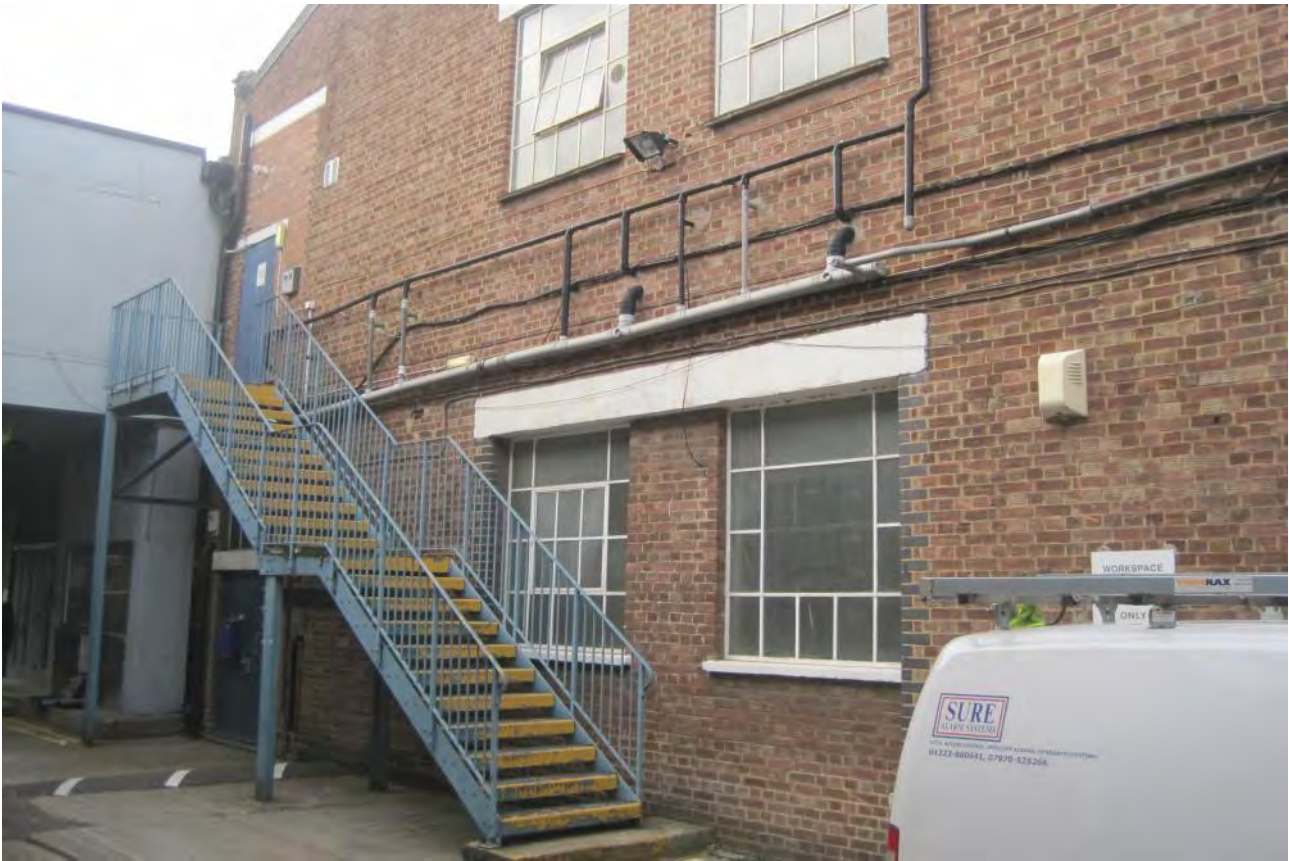
Photo No 21: External fire escape staircase to Building B
