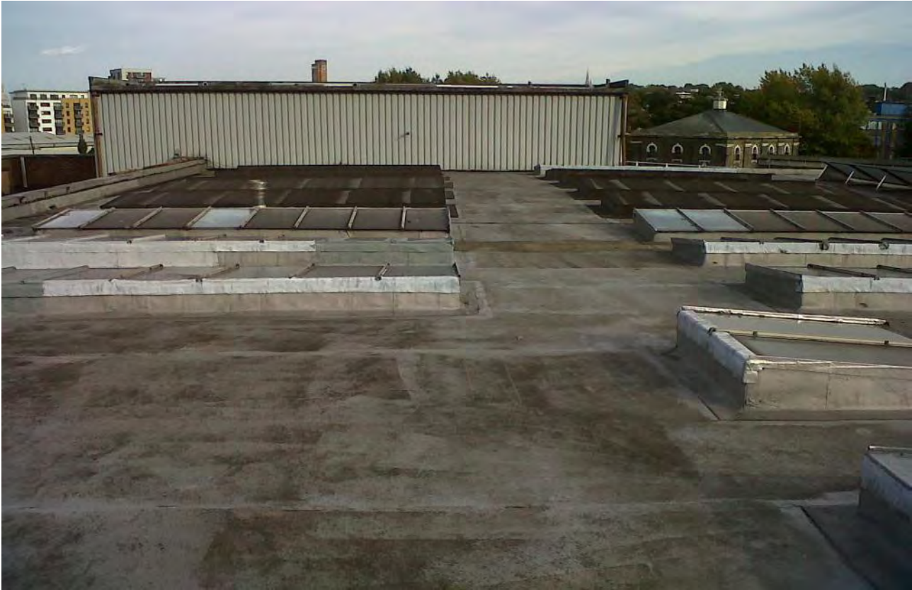
Photo No 4: General view of Building B
