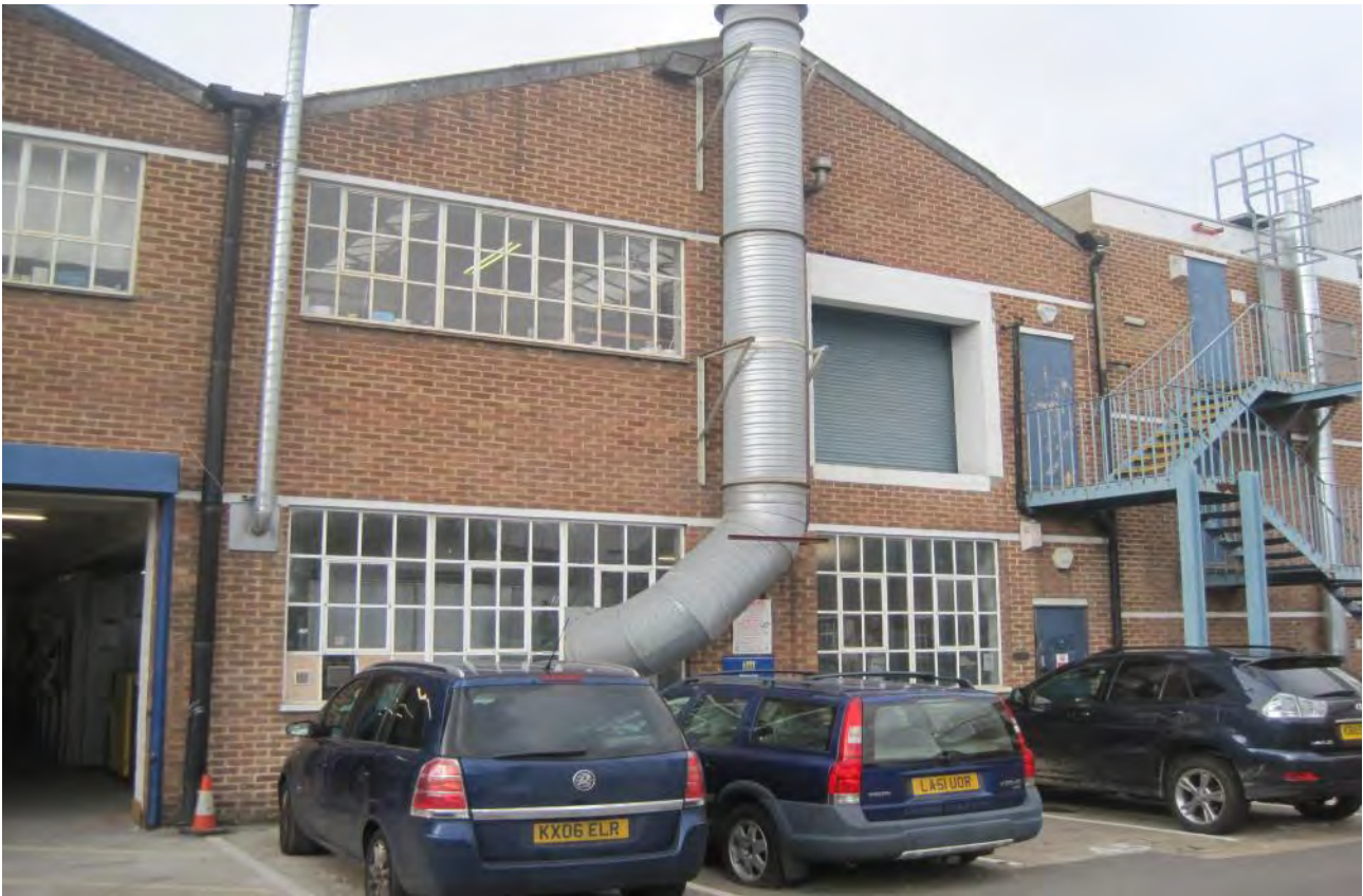
Photo No 11: Rear elevation from main car park of Building A
