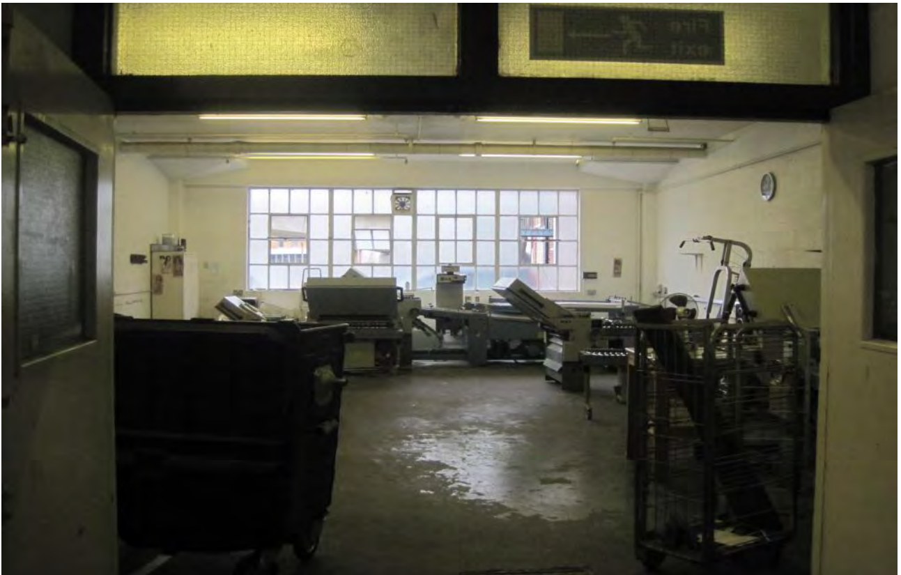
Photo No 16: Ground floor workshop to Building B
