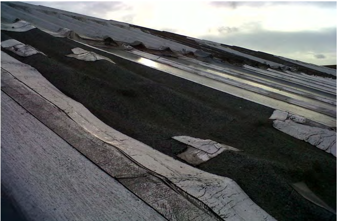
Photo No 6: Patch repairs to Building A
