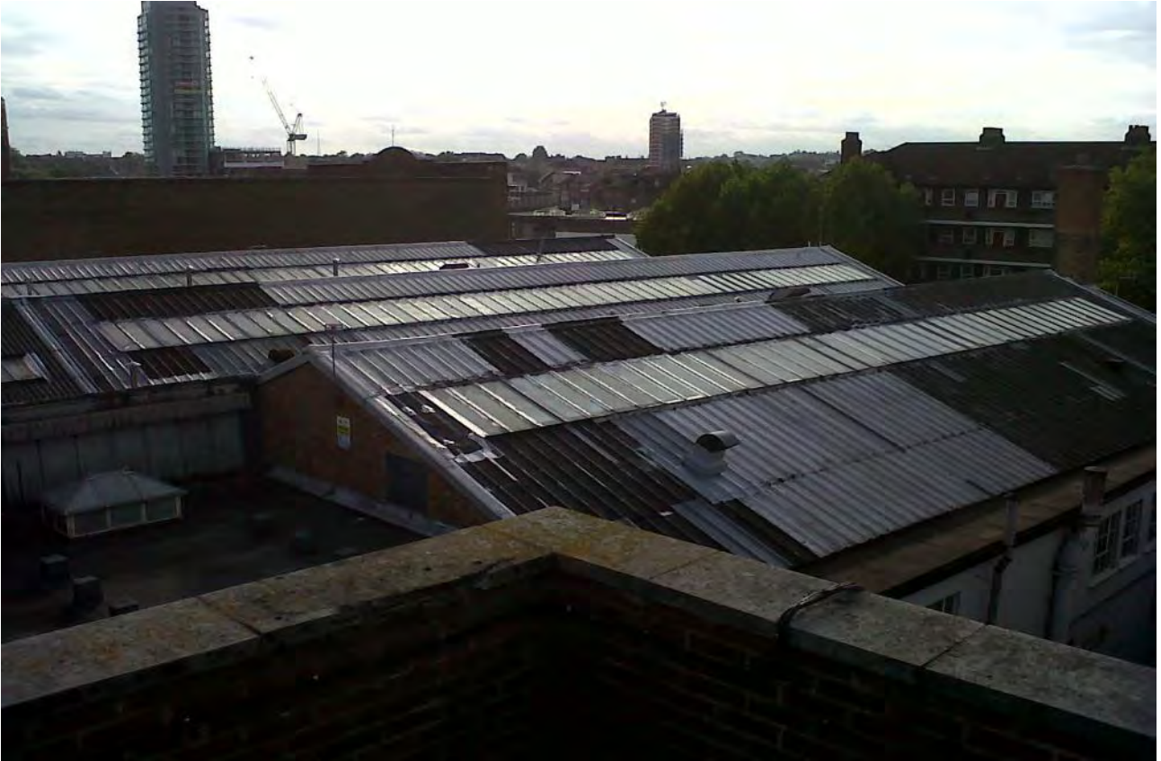
Photo No 1: Front section of Building A
