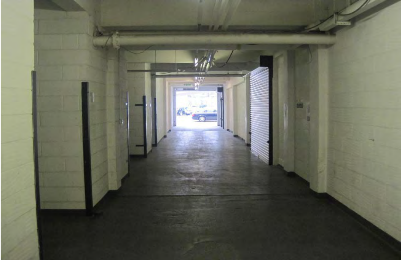
Photo No 7: Central ground floor corridor to Building A
