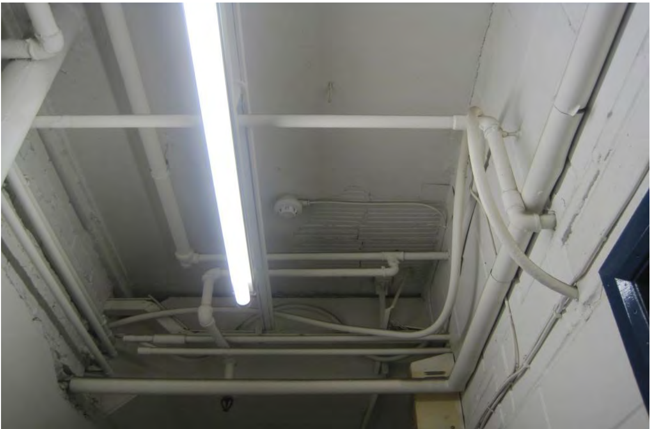
Photo No 18: Exposed pipework to Building B
