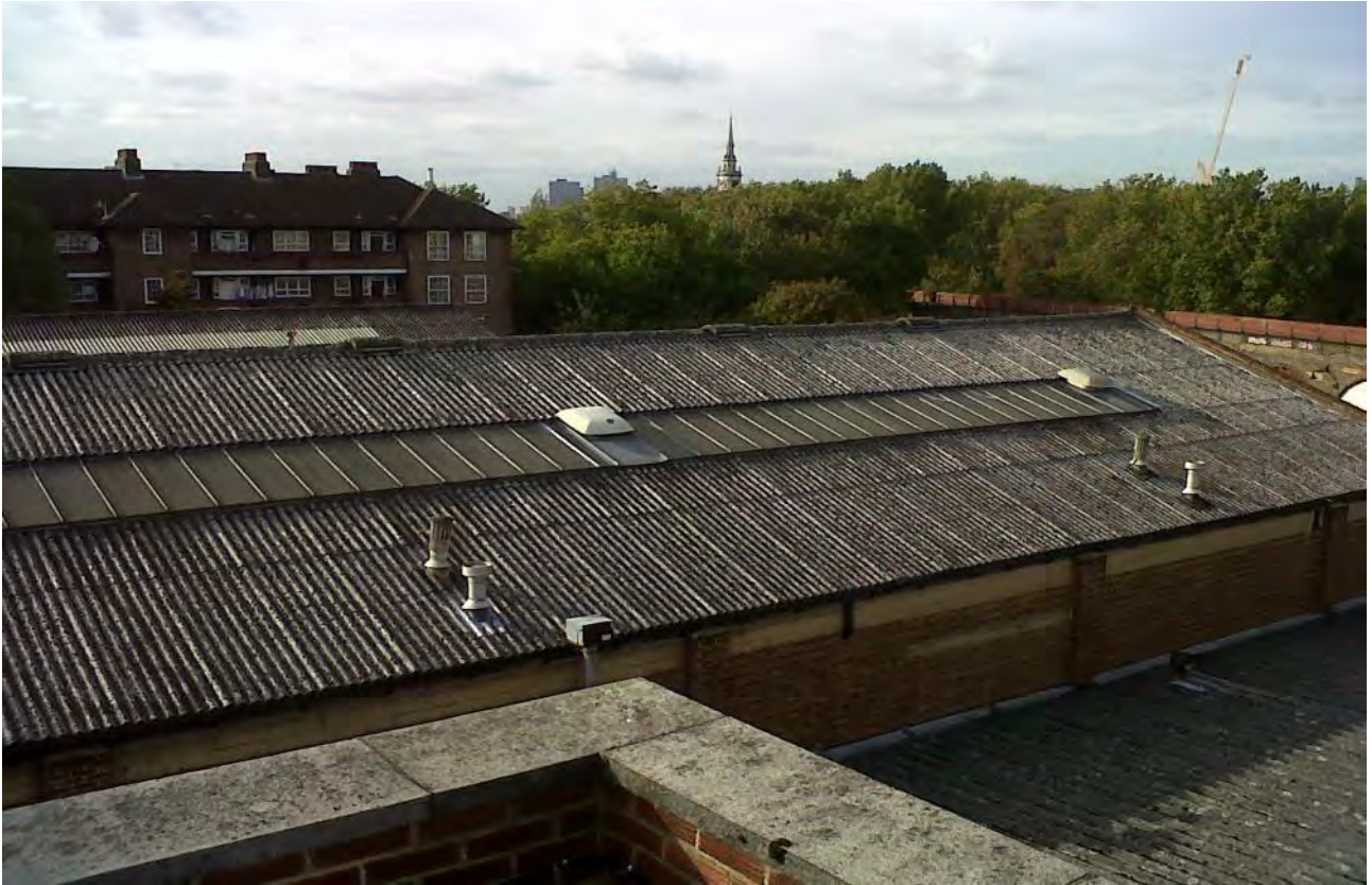
Photo No 5: General view of Building C
