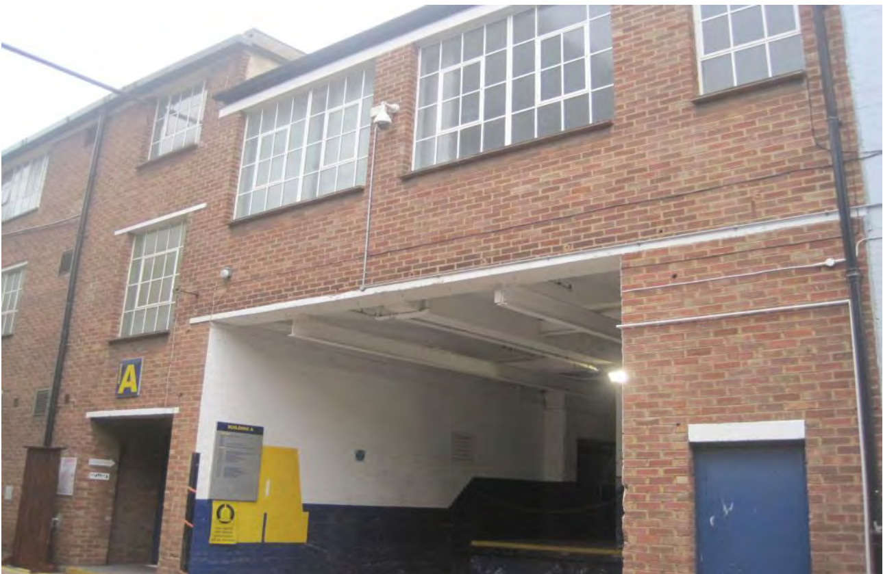
Photo No 10: External wall above loading bay
