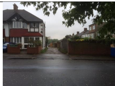
Main access from Rayford Avenue
