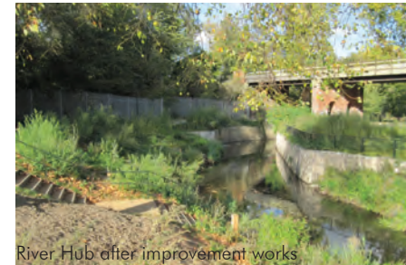
River Hub after improvement works
