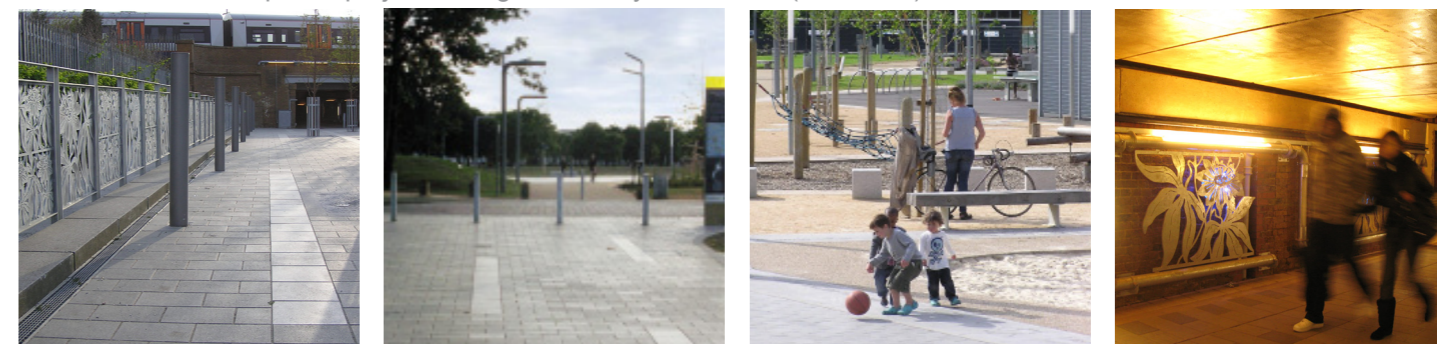
Recent views of completed projects along the Priority Route One (NLL 2007)
