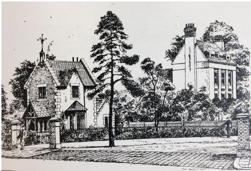
Image 6: Lodge and Villa (no.73) at the north west corner of the Park c 1850s
