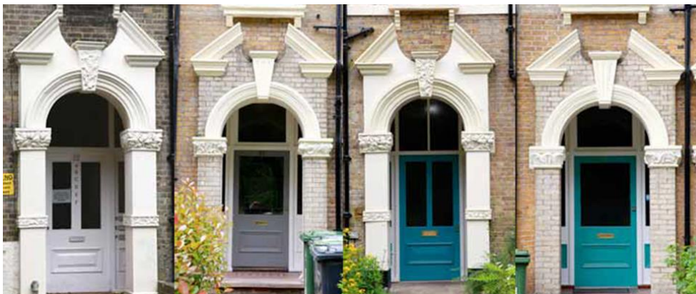
Image 28: Original front doors in recessed porches: Victorian houses
