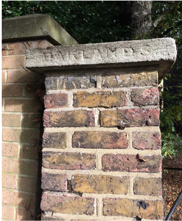
Image 14: Gate pier to the former Oaklands (no.64) north side
