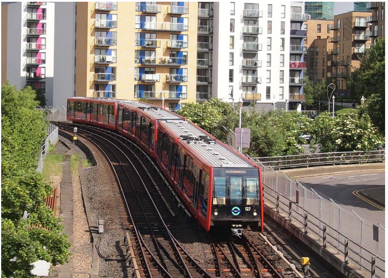
DLR passing existing buildings in the Connington Road Policy Area
