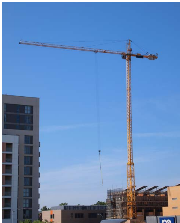
New development near Cornmill Gardens
