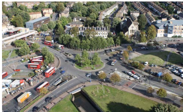
Existing roundabout to be replaced by mixed use development
