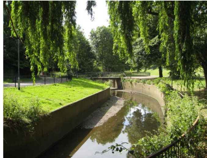
Railings, river in concrete culvert/channel - the hub
