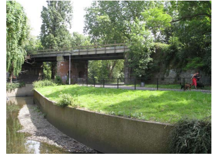
Steep banks to the river - the hub
