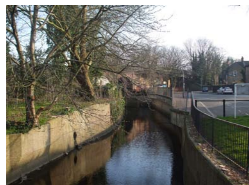
Middle reach - toe boards and shelves
