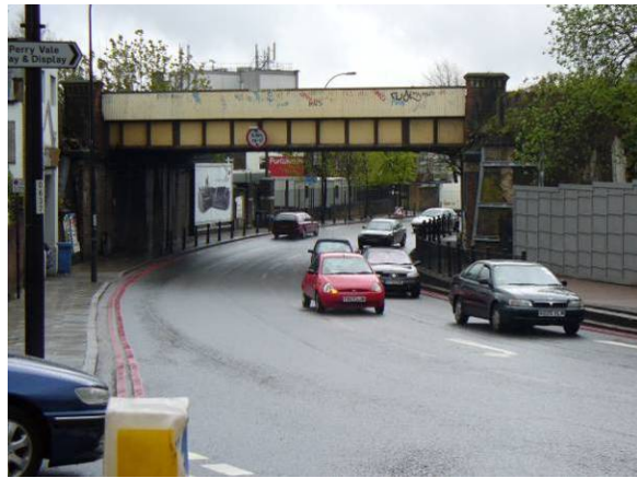
The railway bridge on Waldram Crescent
