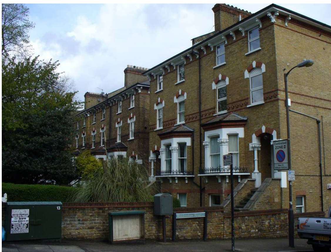
Semi-detached villas on London Road exhibiting the characteristic details of yellow London stock brick with stucco and red brick detailing, three storey construction, with basements and shallow pitched hipped roofs of Welsh slate
