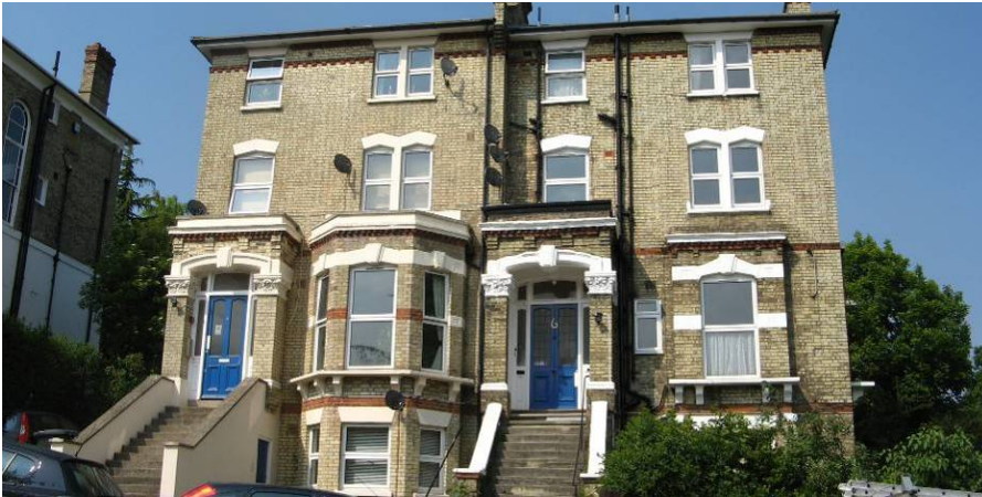
Two houses at Manor Mount that have lost character through the replacement of traditional timber sash windows with uPVC units
