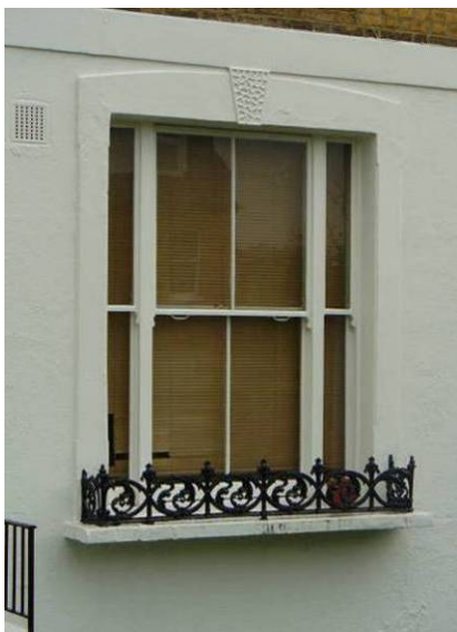
Above left: Detail of tripartite sash window with cast metal window guard at Devonshire Road.
