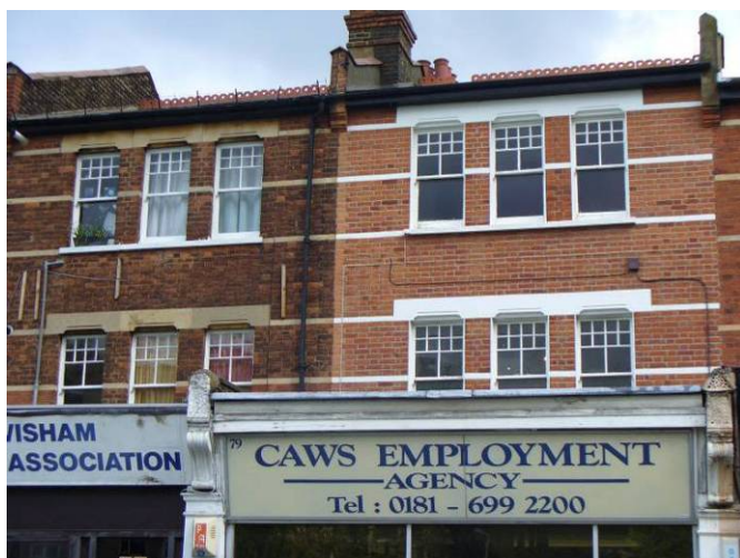
Above right: First and second floor windows above shops at Dartmouth Road with elaborately decorated widow hoods, polychrome brick window arches and well preserved chimney stacks above.
