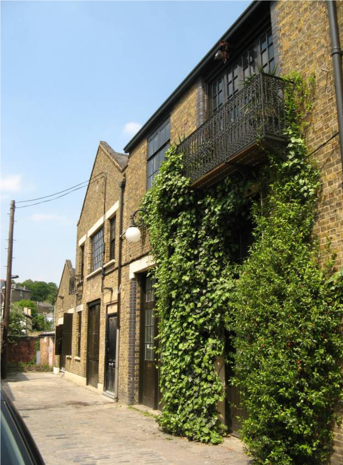
Redevelopment of historic warehousing for Live/Work units at Havelock Walk
