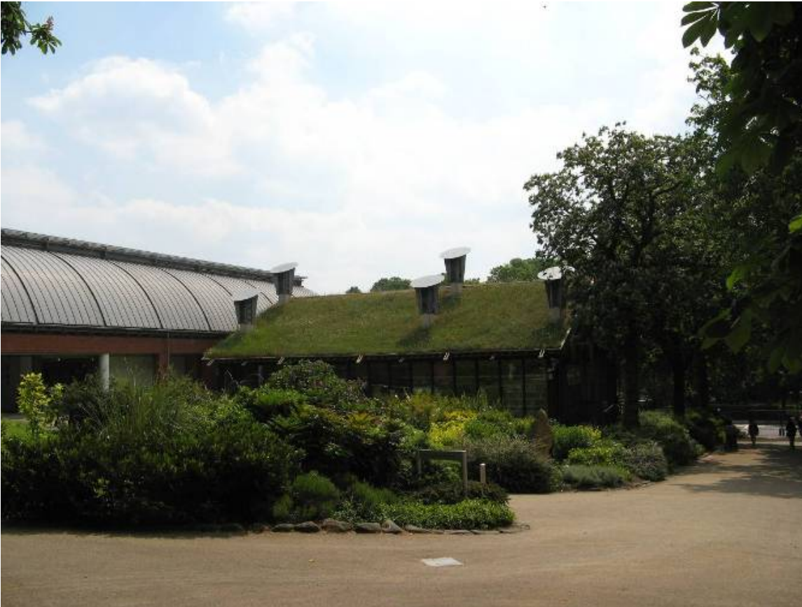
The CUE Building at the Horniman Museum was designed to make a positive contribution to both the natural and built environment
