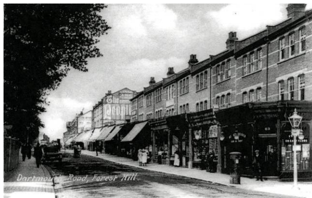
An early 20 th century view looking north along Dartmouth Road
