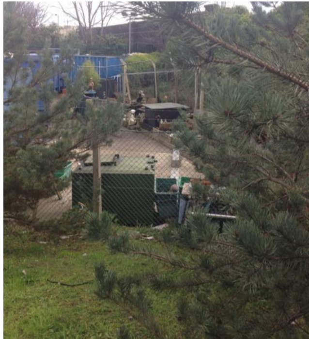
Figure 5-4: Landmann Way Waste Reception Centre, taken from SELCHP
