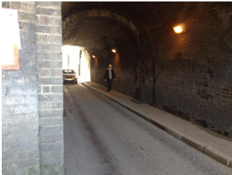
Figure 3-9: Single lane carriageway through railway tunnel on Cold Blow Lane
