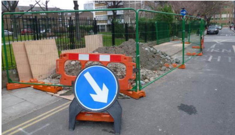
Figure 2-5: DH trench spoil area
