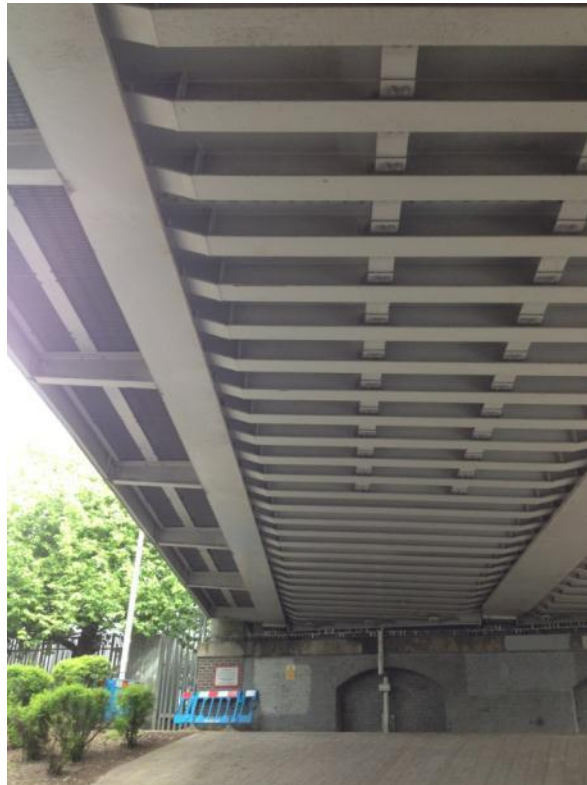
Figure 3-7: Underside of Surrey Canal Bridge structure
