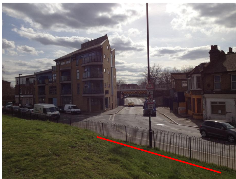
Figure 3-17: Proposed area for pipe installation to the edge of Folkestone Gardens (looking towards Sanford Street)
