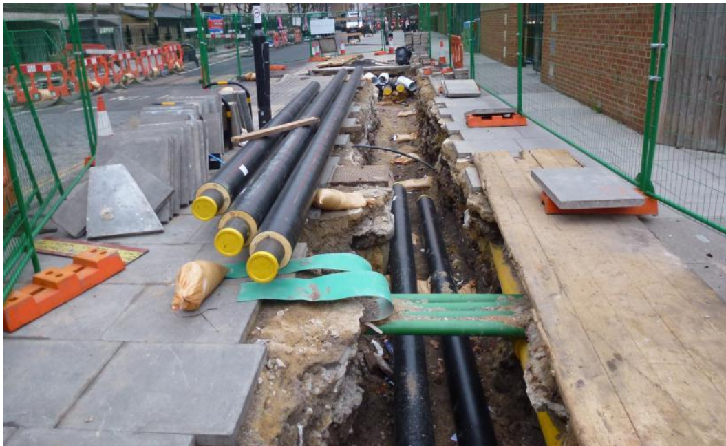
Figure 2-4: DH trench example
