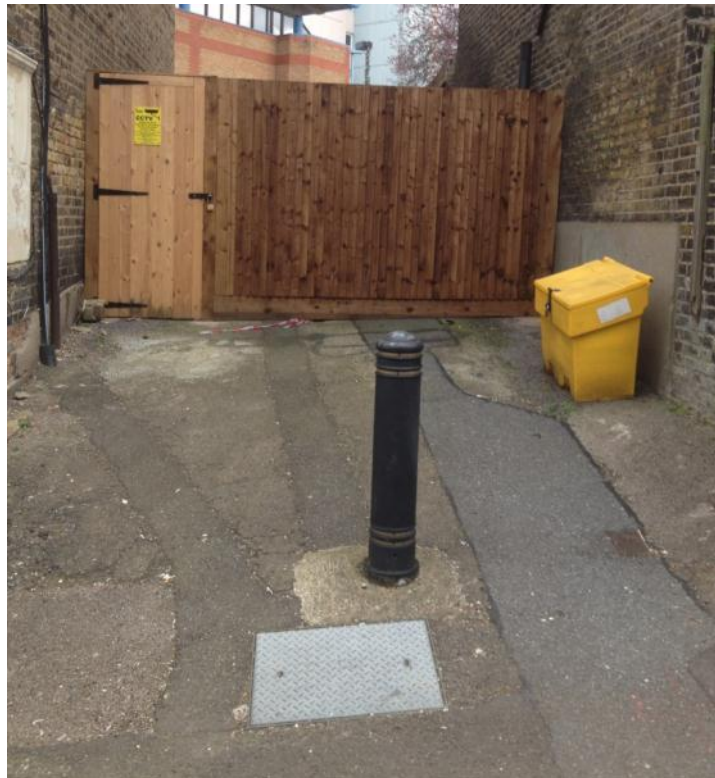
Figure 5-7: Passageway from Laurie Grove through to Education Building (taken from Laurie Grove)
