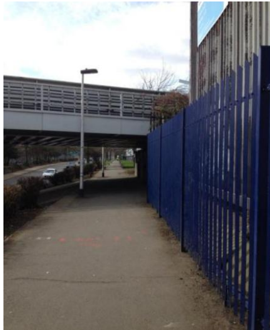
Figure 3-3: Cycle path to north of Surrey Canal Road
