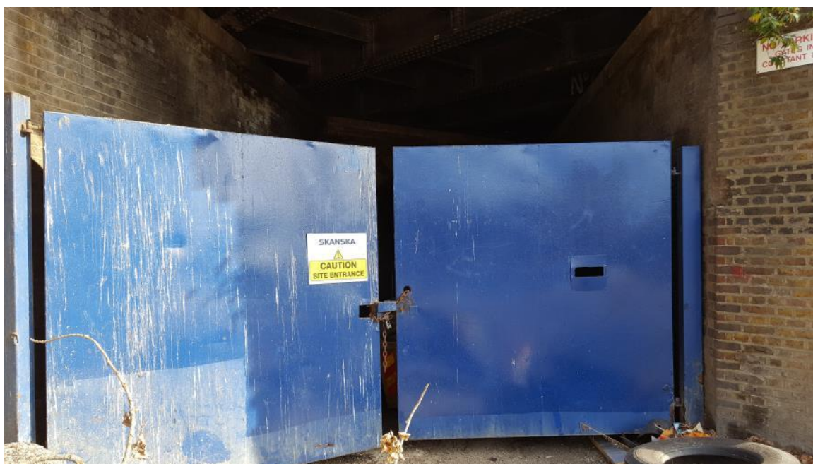
Figure 7-1: Locked entrance to Canal Approach on Surrey Canal Road
