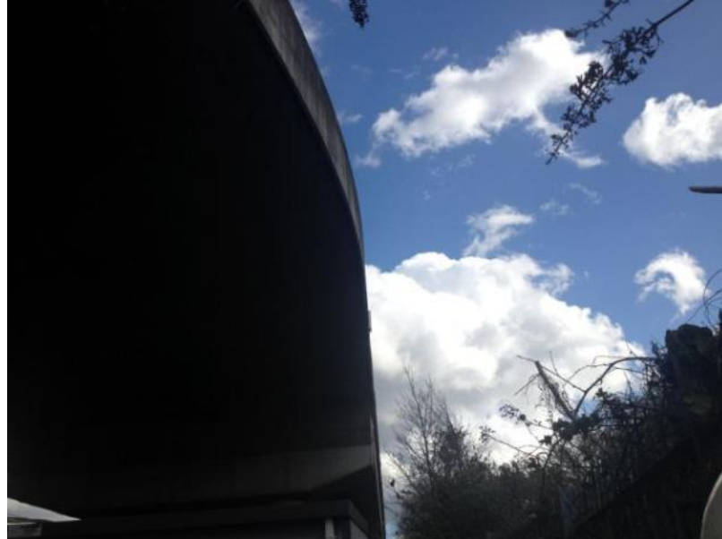
Figure 9-2: Underside of ramp within SELCHP - pipes to be suspended from here
