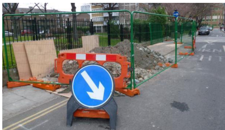
Figure 3-3: DH trench spoil area
