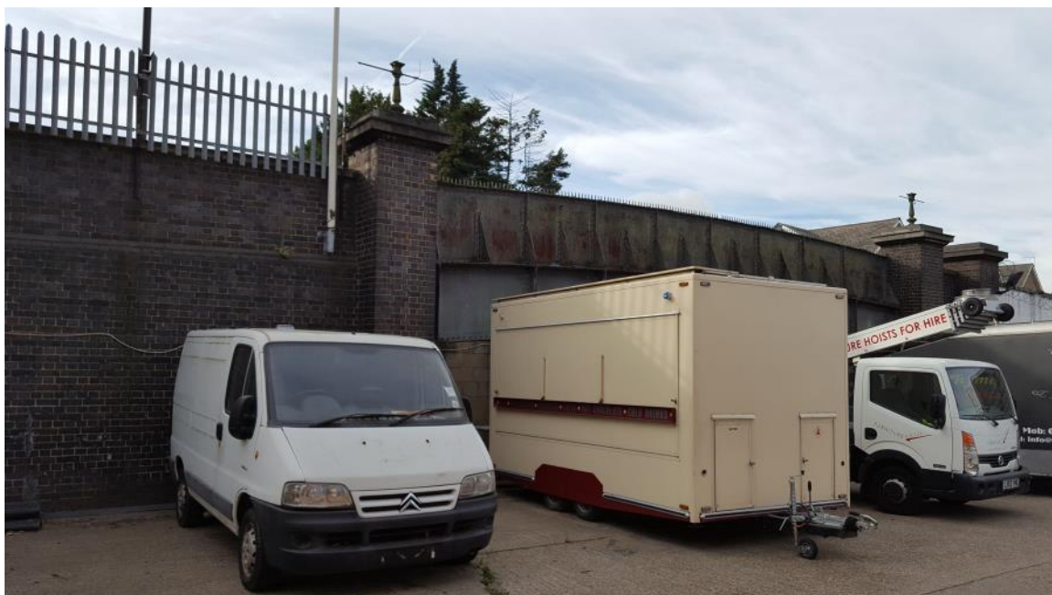
Figure 7-5: Evelyn Street road bridge southbound side - taken from Selfstore car park
