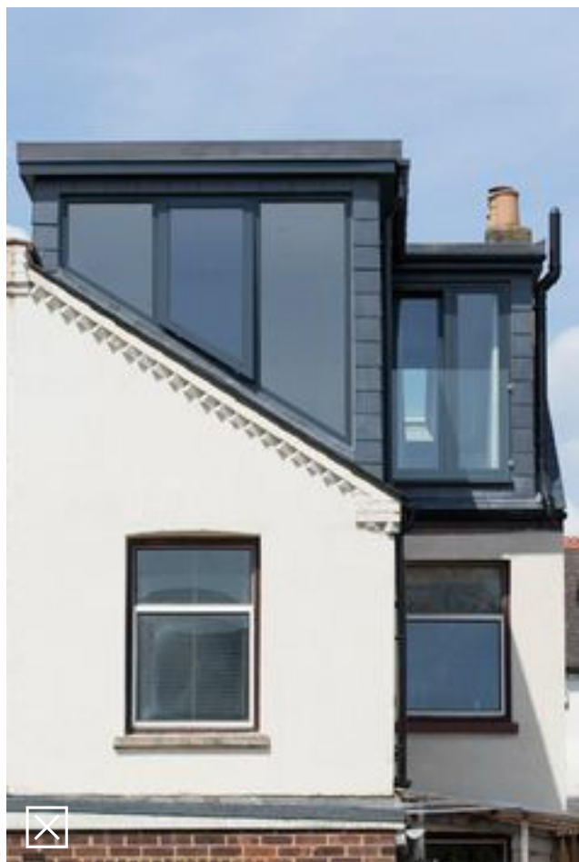
Fig 5.28: Unacceptable as the extension is overbearing and dominates the original property
