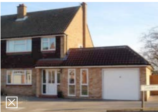
Fig 4.16: Unacceptable because the side extension is more than half the width of original house and is not set back from original frontage
