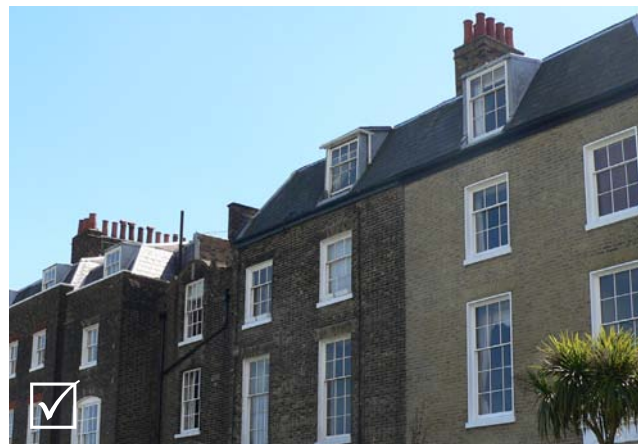
Fig 5.11: Acceptable due to its slender, subordinate form and alignment with the elevation below
