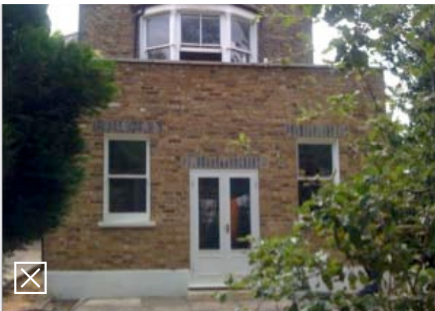
Fig 4.5: Unacceptable because the single storey rear extension is incongruous. This negatively impacts on the integrity of the original building form because it is too high, impacting on the first floor rear bay window
