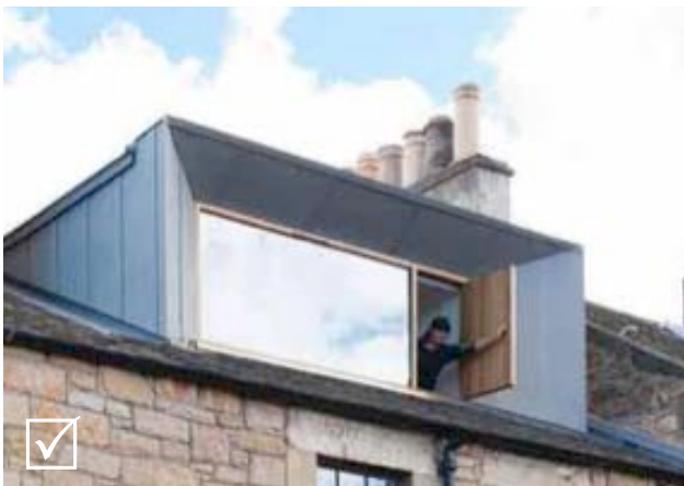
Fig 5.17: Acceptable due to its innovative design, high quality materials and its location set in from the eaves, ridge and sides
