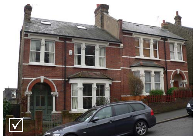
Fig 5.5: Acceptable - roof lights are discrete, subordinate features on the roof, flush within the roof, aligned with the elevation below and clear from roof ridge
