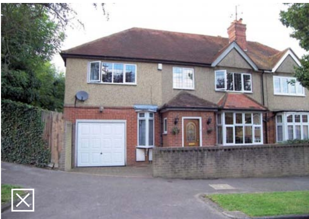
Fig 4.19: Unacceptable as it is not subordinate and the width is more than half of the existing building
