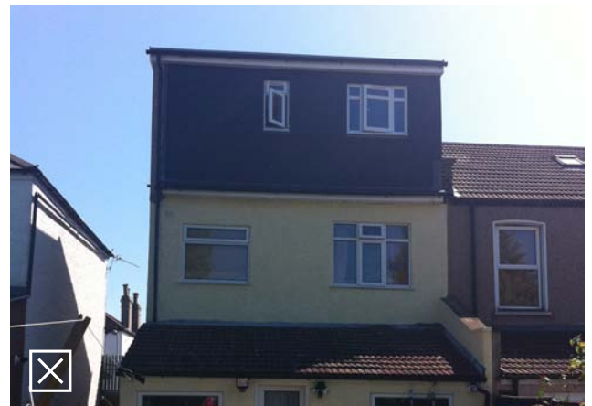
Fig 5.18: Unacceptable owing to the obtrusive nature of the extension. This obliterates the eaves, ridge or sides
