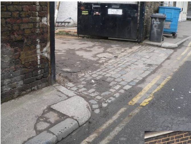
Left: Historic granite setts and kerb at Greenwich MOT
