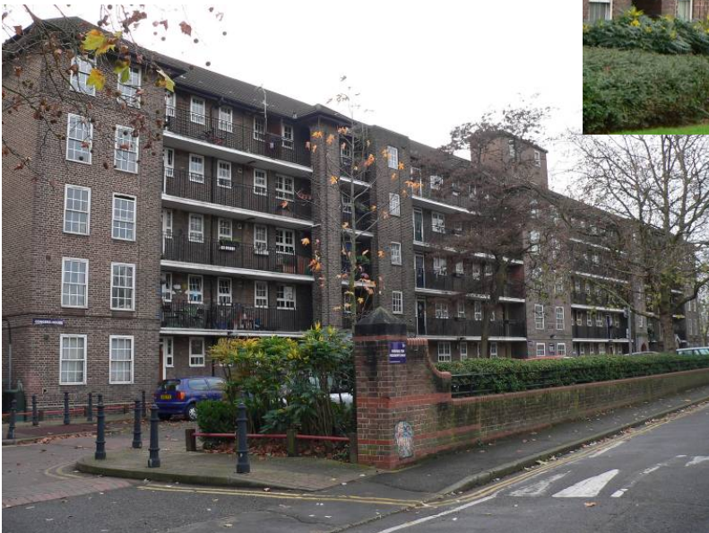
The three different types of blocks at the Crossfield Estate. Clockwise from top left: Castell House of the group of inter-war houses south of the railways; Farrer House, the last of the blocks to be built in 1949, and Congers House at Bronze Street built in the late 1940s.
