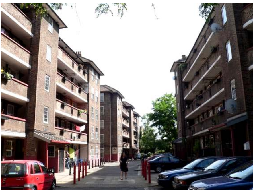
The central cul-de-sac, formerly Addey Street, which was laid out in the mid 19 th century.
