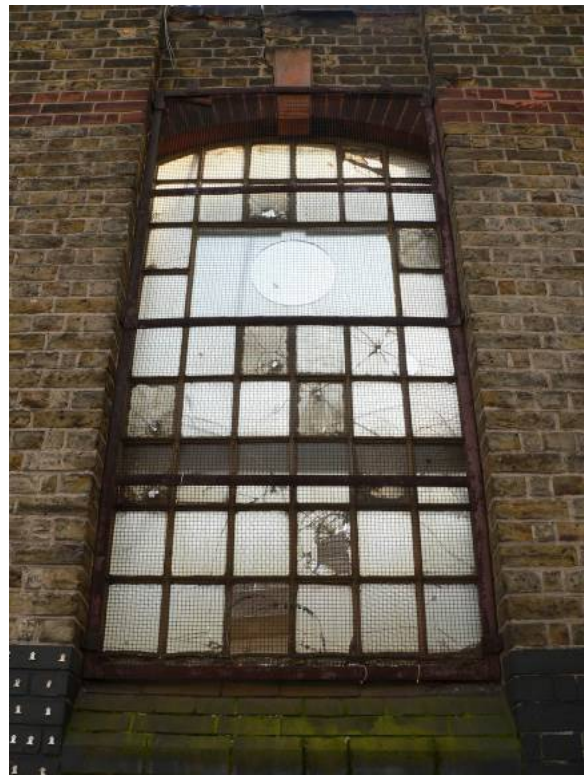
Building materials and details of the area I: Clockwise from the top: Yellow London stock brick, red brick and Terracotta have been combined at the APT Building, 6 Harold Wharf; Victorian cast-iron windows at the ancillary industrial building at 6 Harold Wharf; The impressive stone faced pilaster at the railway bridge, a remainder of the Victorian predecessor of the present bridge.
