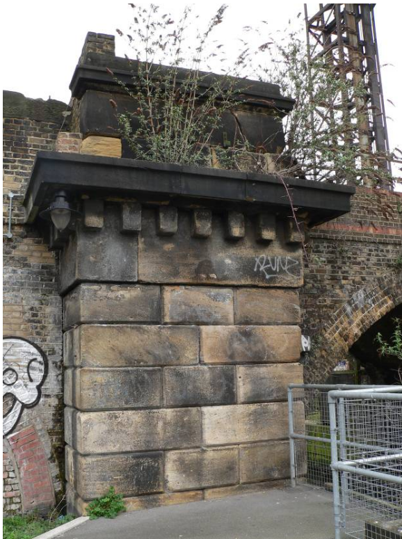
Building materials and details of the area I: Clockwise from the top: Yellow London stock brick, red brick and Terracotta have been combined at the APT Building, 6 Harold Wharf; Victorian cast-iron windows at the ancillary industrial building at 6 Harold Wharf; The impressive stone faced pilaster at the railway bridge, a remainder of the Victorian predecessor of the present bridge.
