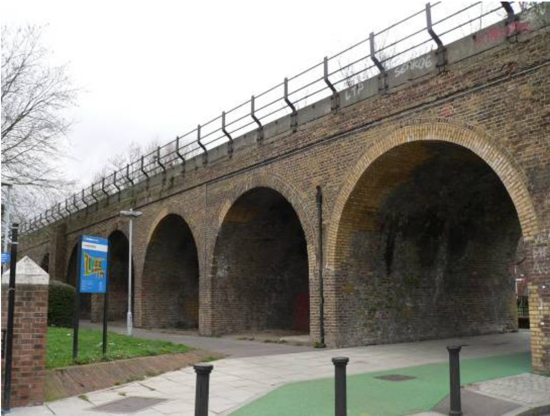
A section of the listed 1838 railway viaduct
