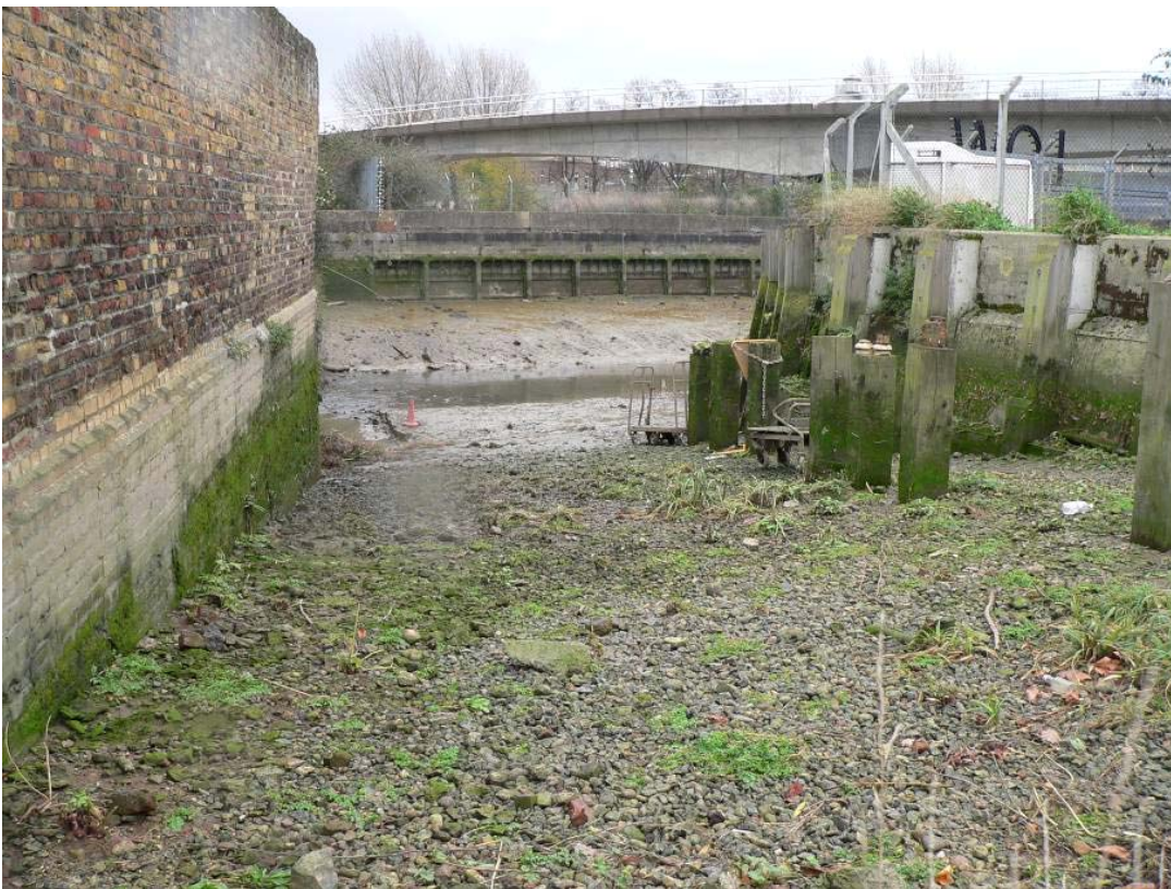
The beach at the Creekside Centre, formerly a small dock to the Transco Inlet. The beach was created in 2002 and left for natural colonisation as innovative flood defence.
