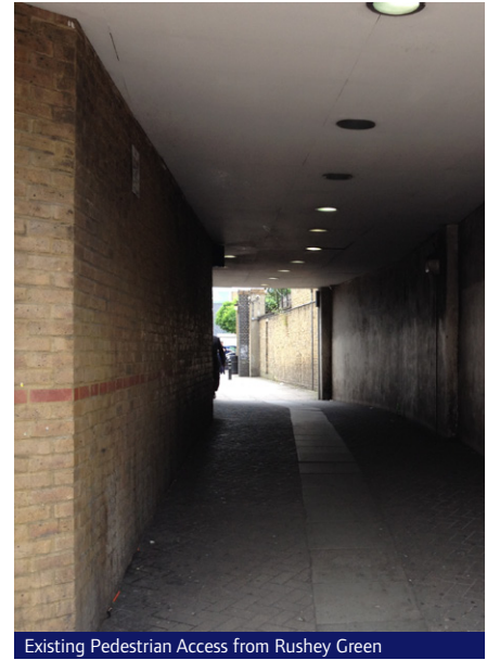
Existing Pedestrian Access from Rushey Green
