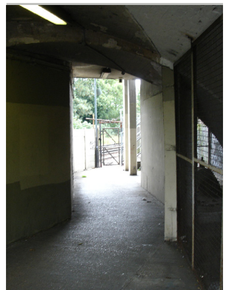
Underpass from the Stations to the Wickes Site
