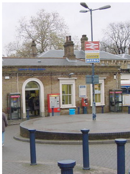
Catford Bridge Station - Doggett Road Entrance
