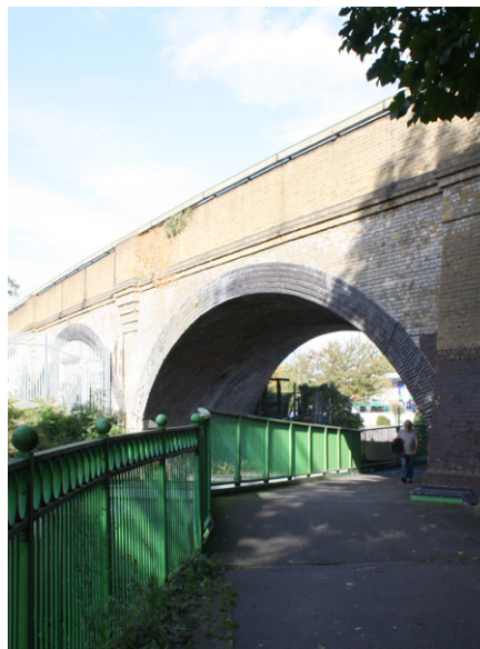
Pedestrian Link Under Viaduct
