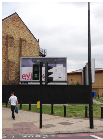
View of Plassy Road Site from Bromley Road
