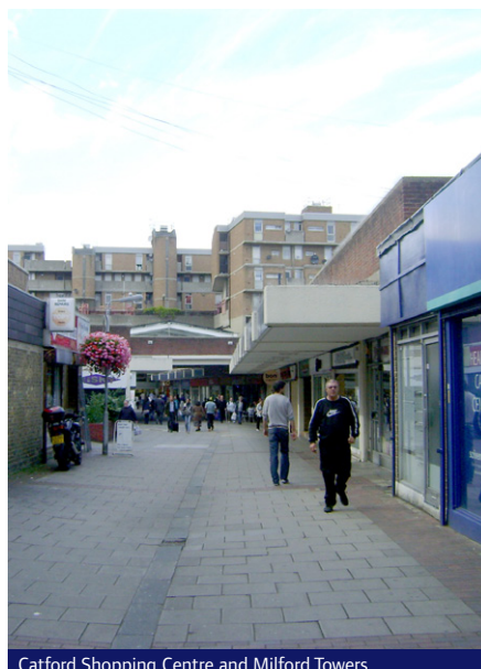
Catford Shopping Centre and Milford Towers
