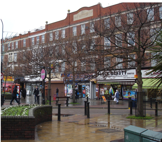
Secondary shopping frontage along Catford Broadway
