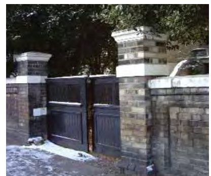
A historic front boundary treatment
