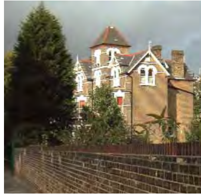
Breakspears Road. Italianate detail and campanile style tower
