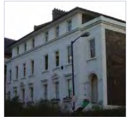
Lea House, Lewisham Way
