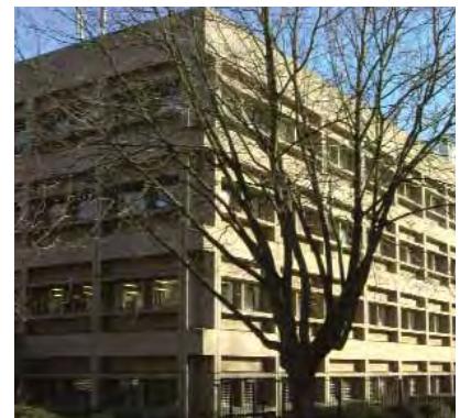
Lewisham College, Breakspears Building, Breakspears Road
