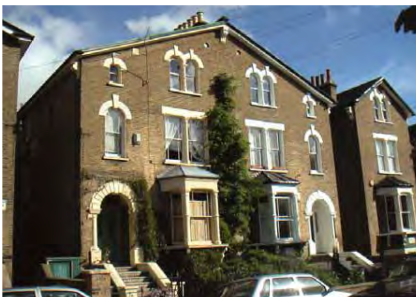
A gable fronted pair of houses in Darling Road
