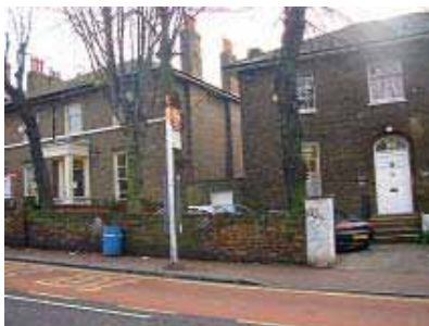
Poor quality modern street furniture and graffiti harm the setting of these listed buildings.
