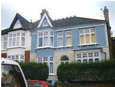
An extreme example of the effect that unsympathetic repainting of a facade can have on the character of a house.
