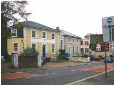
Loss of front gardens and boundary walls to make way for forecourt parking.
