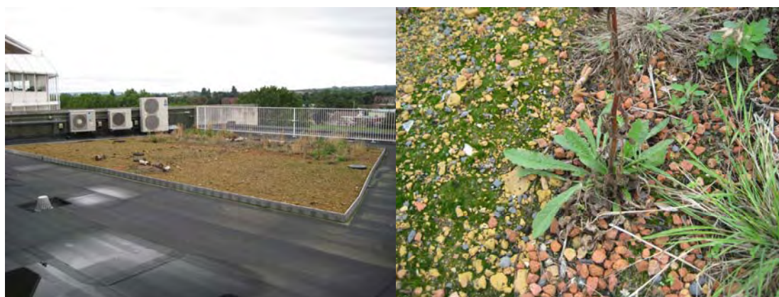
Figure 5.4 Living roofs in Lewisham Town Hall
