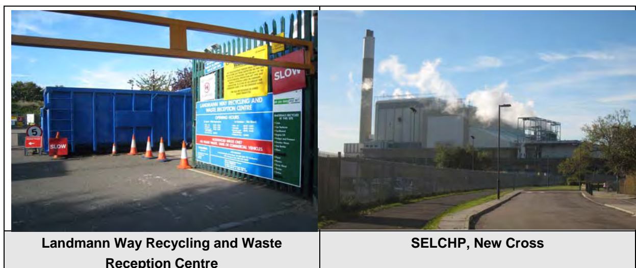
Figure 5.2 Recycling and waste facilities in Lewisham
