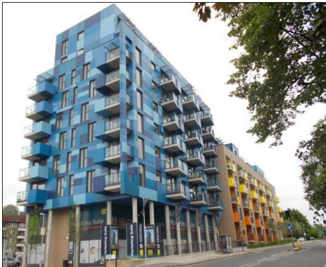
Part of the regeneration of the Heathside and Lethbridge estates, Lewisham, containing private and affordable housing
