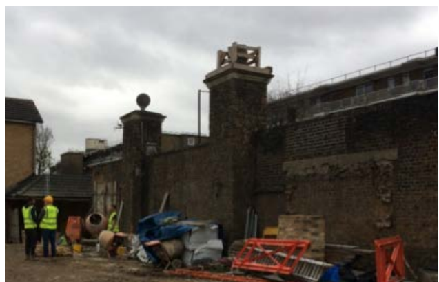
Photo 14: Repairs to Grove Street Wall Image Credit: LB Lewisham
