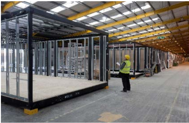
Photo 10: Construction of Fabricated Buildings
