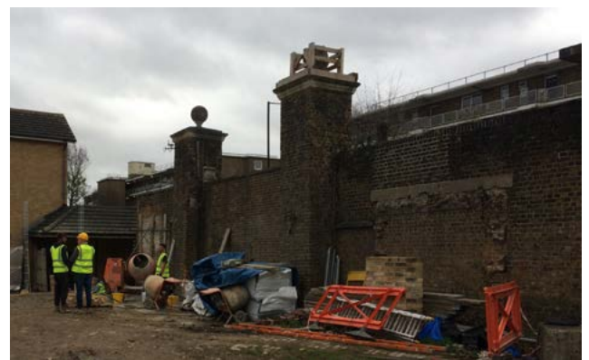
Photo 5: Repairs to Grove Street Wall
