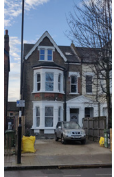
Photo 47: house and garden repaired and cleared
