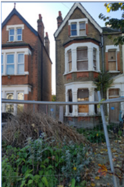
Photo 45: original condition of the house
