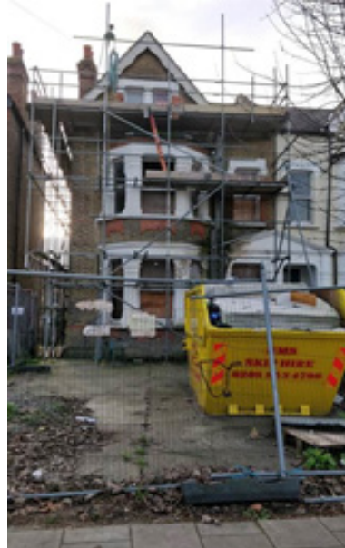
Photo 46: house being repaired after service of section 215 notice
