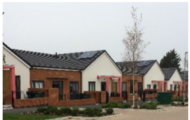
Photo 36: Phase 1 Excalibur Estate Image Credit: LB Lewisham
