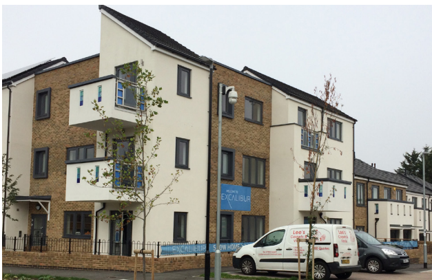
Photo 35: Phase 1 Excalibur Estate Image Credit: LB Lewisham
