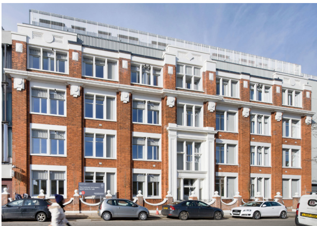
Photo 4: Astra House, Deptford Foundry Image Credit: RCK architects
