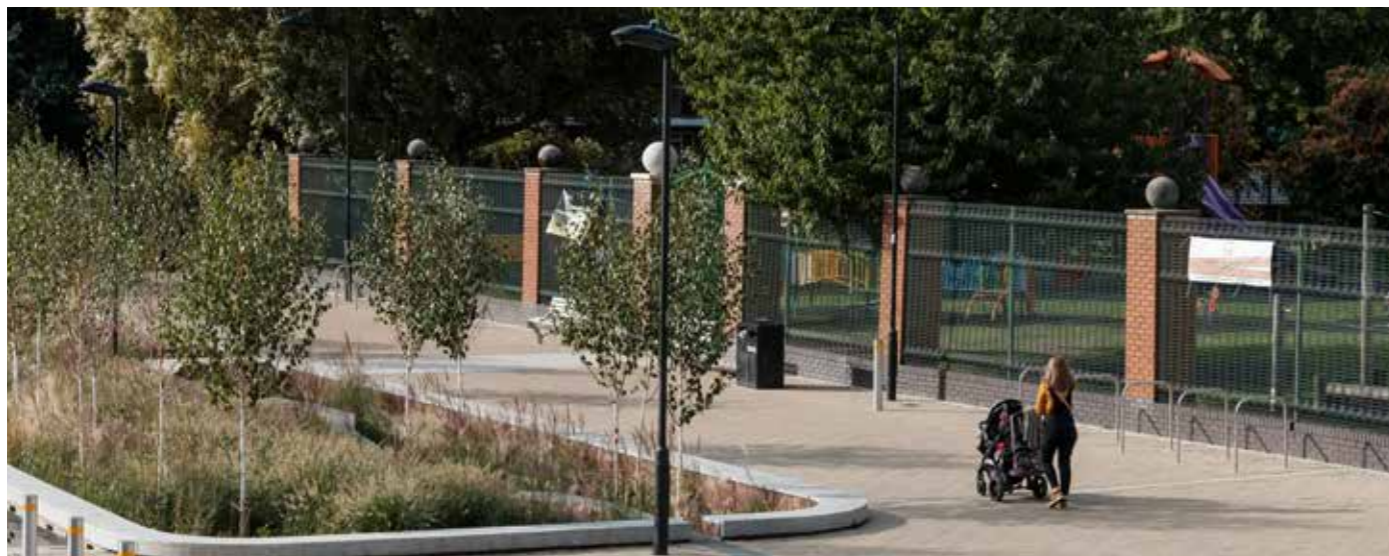
Australia Road, London, where permeable paving provides source control prior to SuDS Basins.
