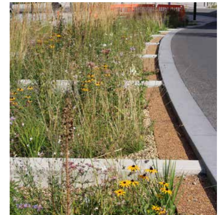
Attractive and wildlife friendly herbaceous planting by Sheffield City Council in a crushed stone bioretention substrate.
