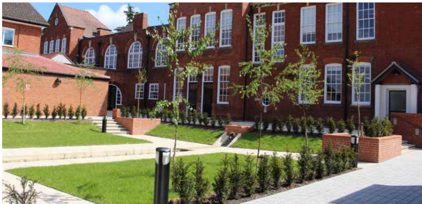
A sunken SuDS courtyard with solar water feature into a formal rill at Bromsgrove Civic Centre.
