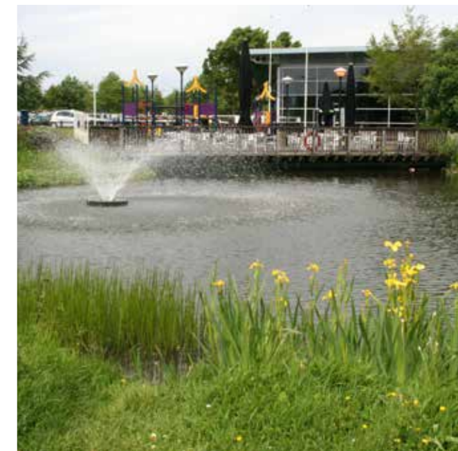
Hopwood Park MSA M42. Wooden terrace and balustrade with wet bench and planted aquatic bench protection to open water.
