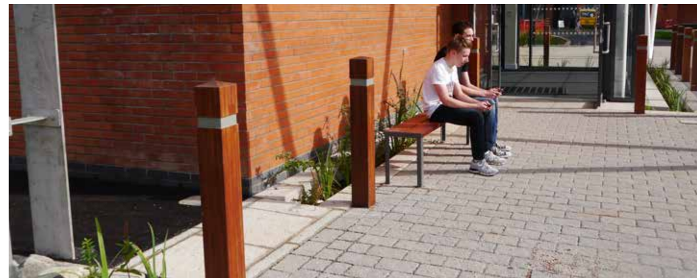
Permeable paving and planted open channels collect runoff from hard surfaces at Bewdley School, Worcestershire.
