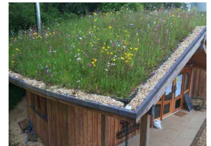
Ruskin Mill Horsely, Glos. Greenroof with gravel edge and rainchain.
