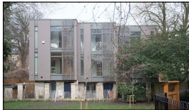
Fig. 169: Backland development in Brockley designed by BPTW Architects (website: www.bptw.co.uk , photography: RCKa)
