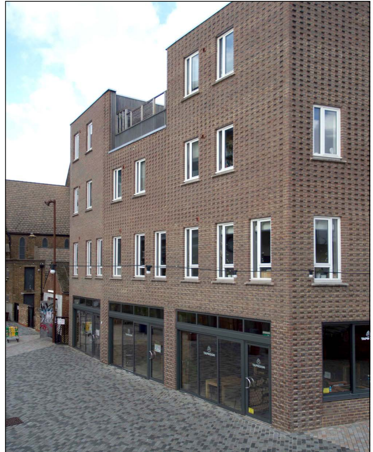
Fig. 74: New homes sit above two commercial spaces in St Paul's House in Deptford designed by Ash Sakula. Access to the homes is kept separate from the commercial units with plenty of opportunity to meet neighbours (website: www.ashsak.com , photography: RCKa)
