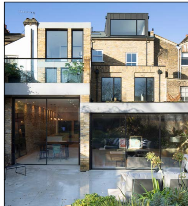
Fig. 71: Coach House in New Cross, designed by Selencky Parsons, is developed by one of the original landowner and delivers three flats and a new house (website: www.selenckyparsons.com , photography: Richard Chivers)
