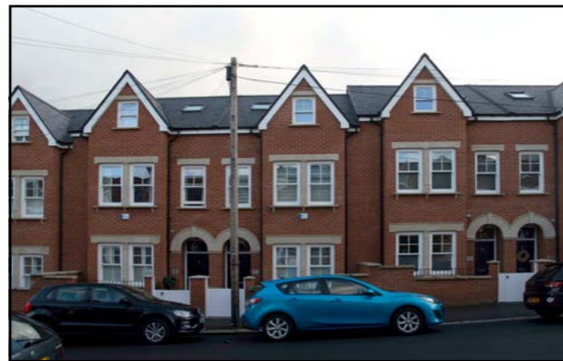
Fig. 107: New homes in Crofton Park designed by Brooks Murray Architects. (website: www.brooksmurray.com , photography: RCKa)
