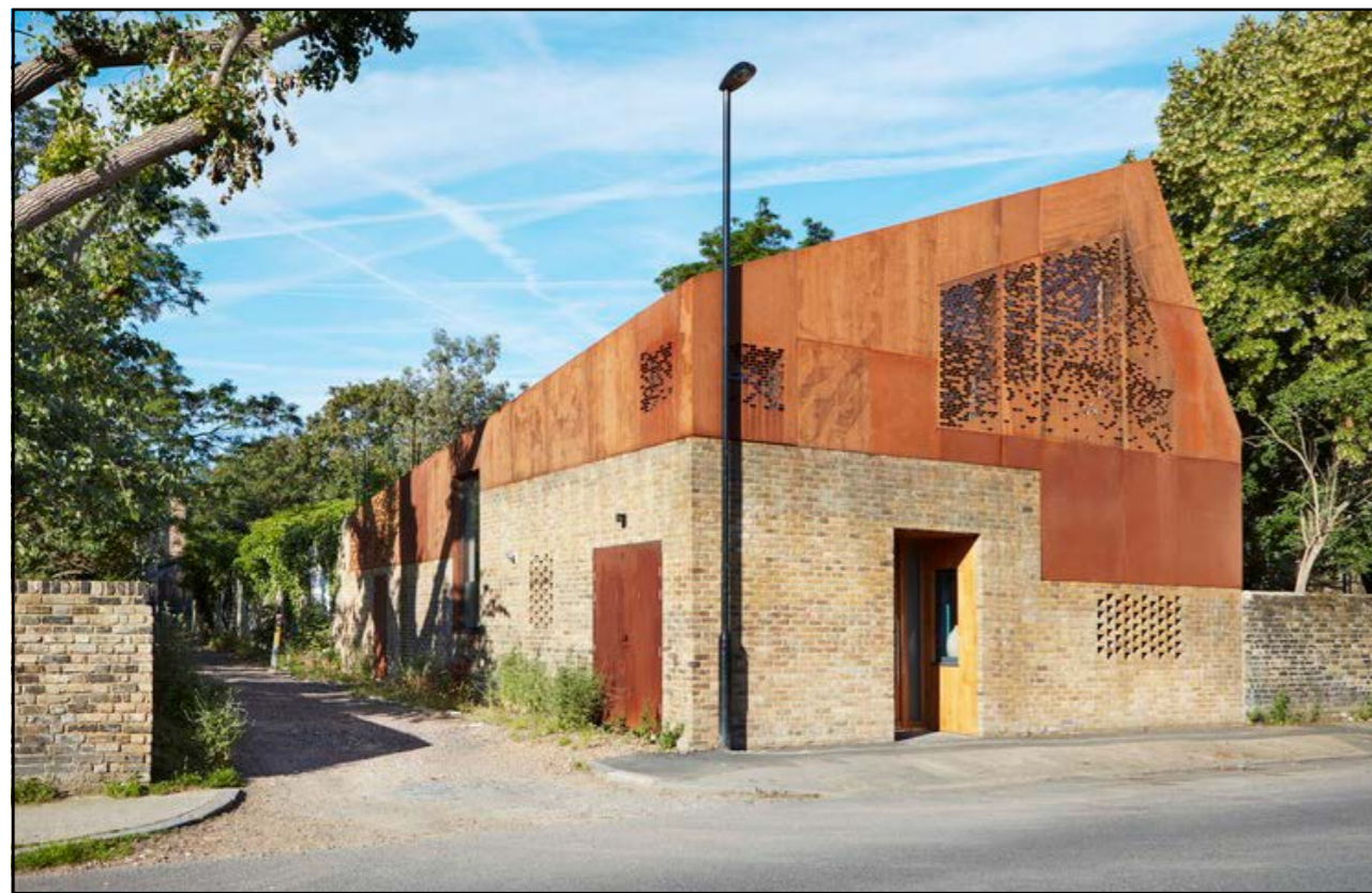
Fig. 125: This new house by Stolon Studio cleverly utilises a site at the entrance to an existing mews to create an attractive family home. The front door is set back from the pavement and ground floor windows use hit-and-miss brickwork to provide privacy. (website: www.stolon.co.uk , photography: Paul Murphy)
