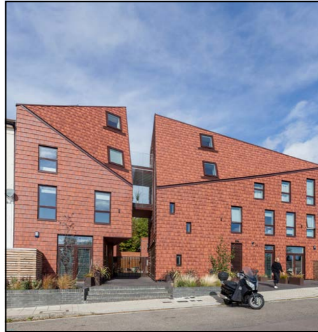
Fig. 106: Kaolin Court by Stolon Studio replaces single-storey workshops and offices with a four-storey development of new homes. The scheme employs a central courtyard which has enabled the use of the whole site. (website: www.stolon.co.uk , photography: Robert Barker)
