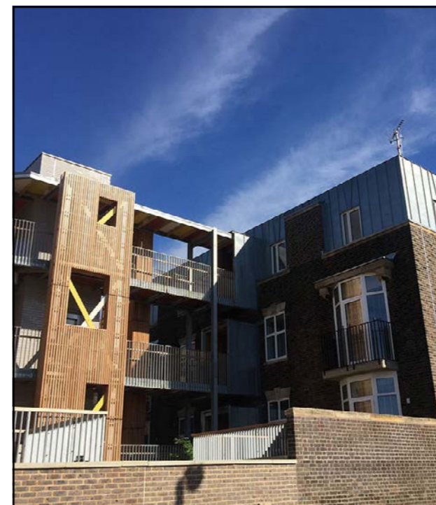
Fig. 159: The refurbishment and vertical extension of St Paul's House in Deptford by Ash Sakula (website: www.ashsak.com , photography: Ash Sakula)
