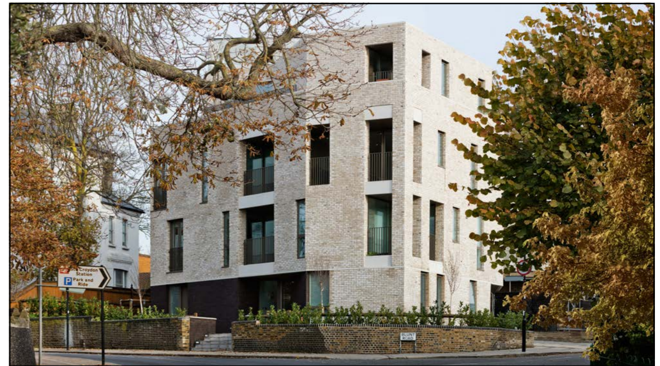
Fig. 138: This development in Croydon by OB Architecture creates a striking, high-density residential development on a prominent corner, with a building taller than its neighbours. (website: obarchitecture.co.uk , photography: Martin Gardner)
