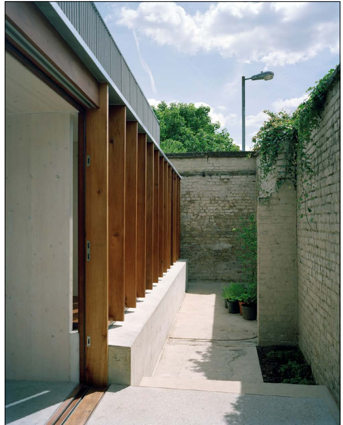
Fig. 88: Strange House designed by Hugh Strange Architects cleverly slots a new family home onto a backland infill site in Deptford. (website: www.hughstrange.com, photography: David Grandorge)
