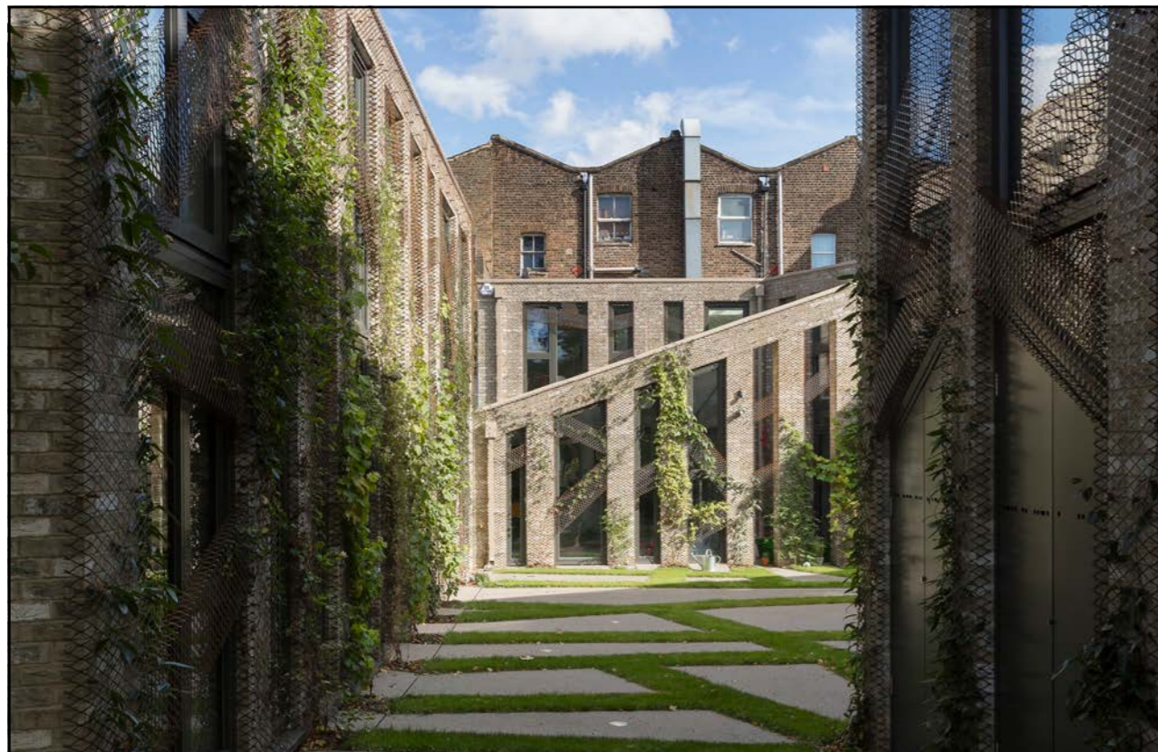
Fig. 34: Access into Forest Mews, designed by Stolon Studio, is via a private road which allows soft landscaping to be integrated into the vehicular access (website: www.stolon.co.uk, photography: Robert Barker)
