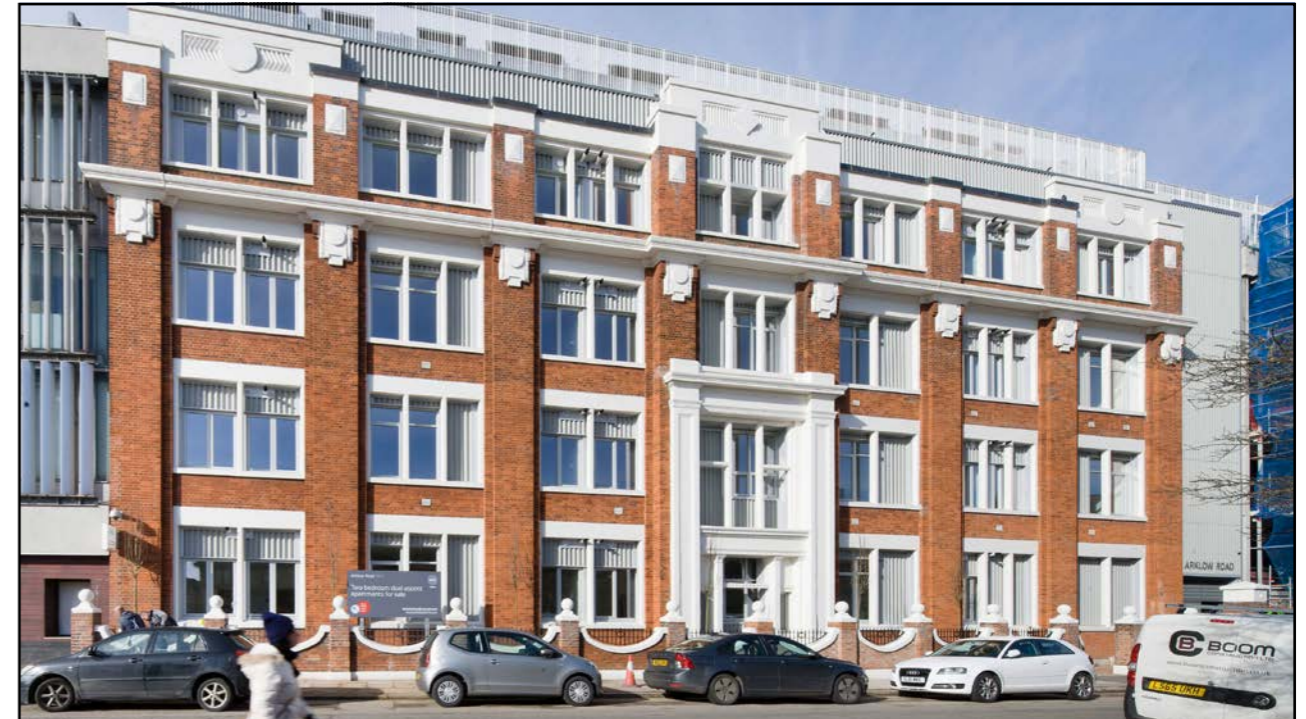
Fig. 156: The refurbishment and vertical extension of Astra House in New Cross by RCKa provides new dual-aspect residential accommodation through the intensification of a formal commercial building. (website: www.rcka.co.uk , photography: Jakob Spriestersbach)
