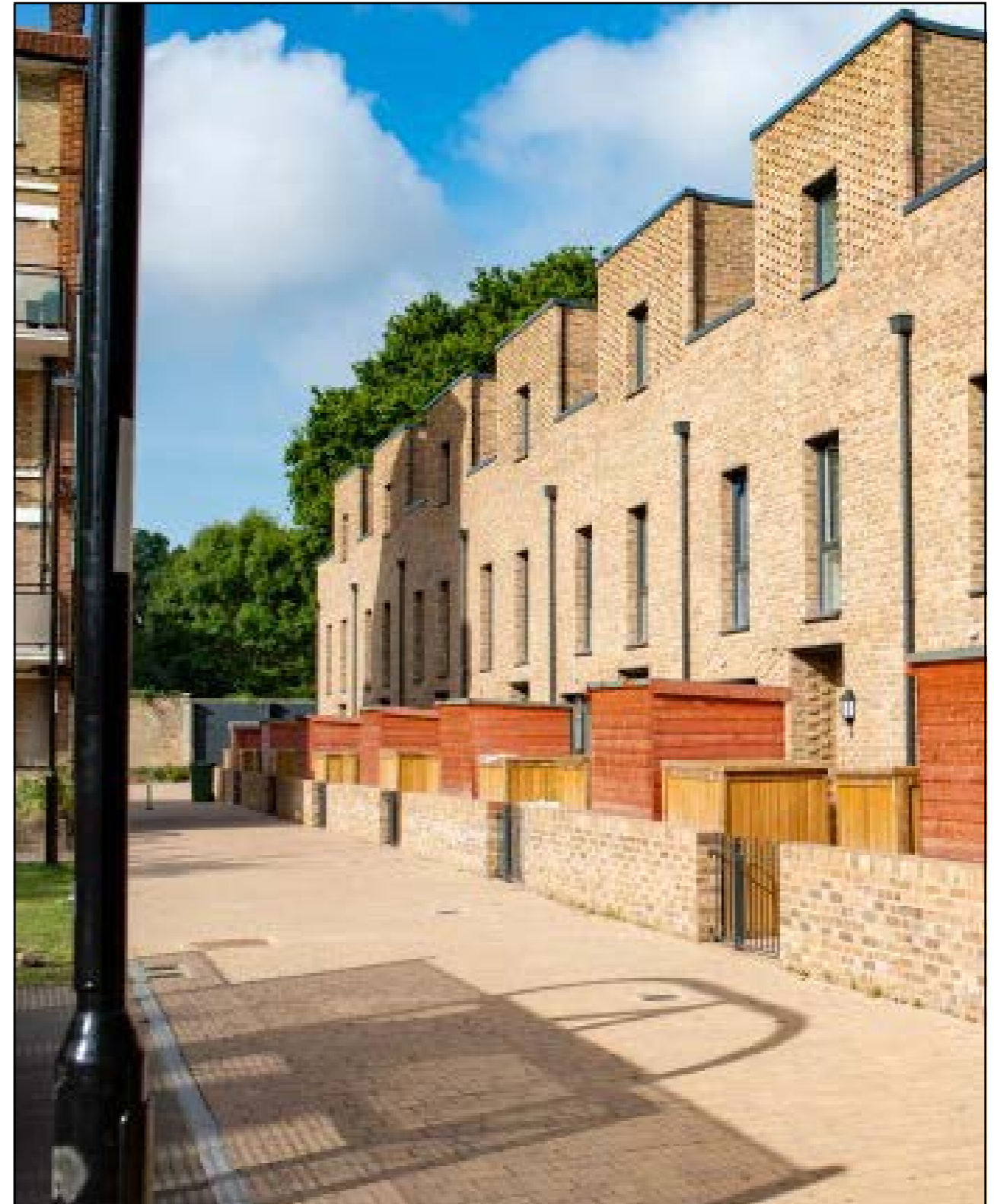
Fig. 16: New homes at Longfield Crescent in Forest Hill designed by Pollard Thomas Edwards Architects. (website: www.pollardthomasedwards.co.uk )
