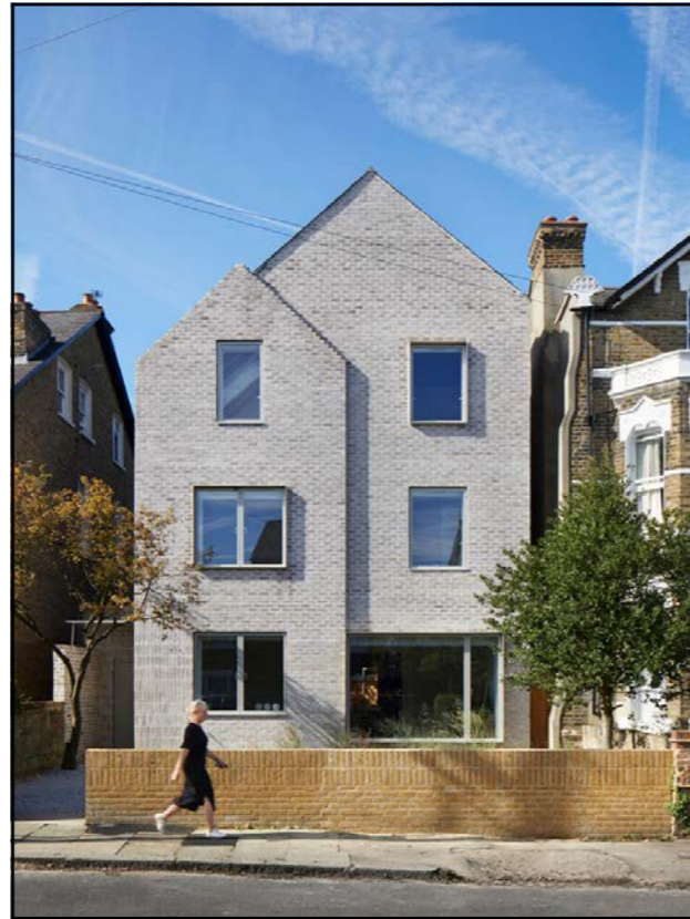
Fig. 181: Vertical extension and recladding of an existing house following the principles of street infill development. Designed by alma-nac (website: www.alma-nac.com, photography: Jack Hobhouse).
