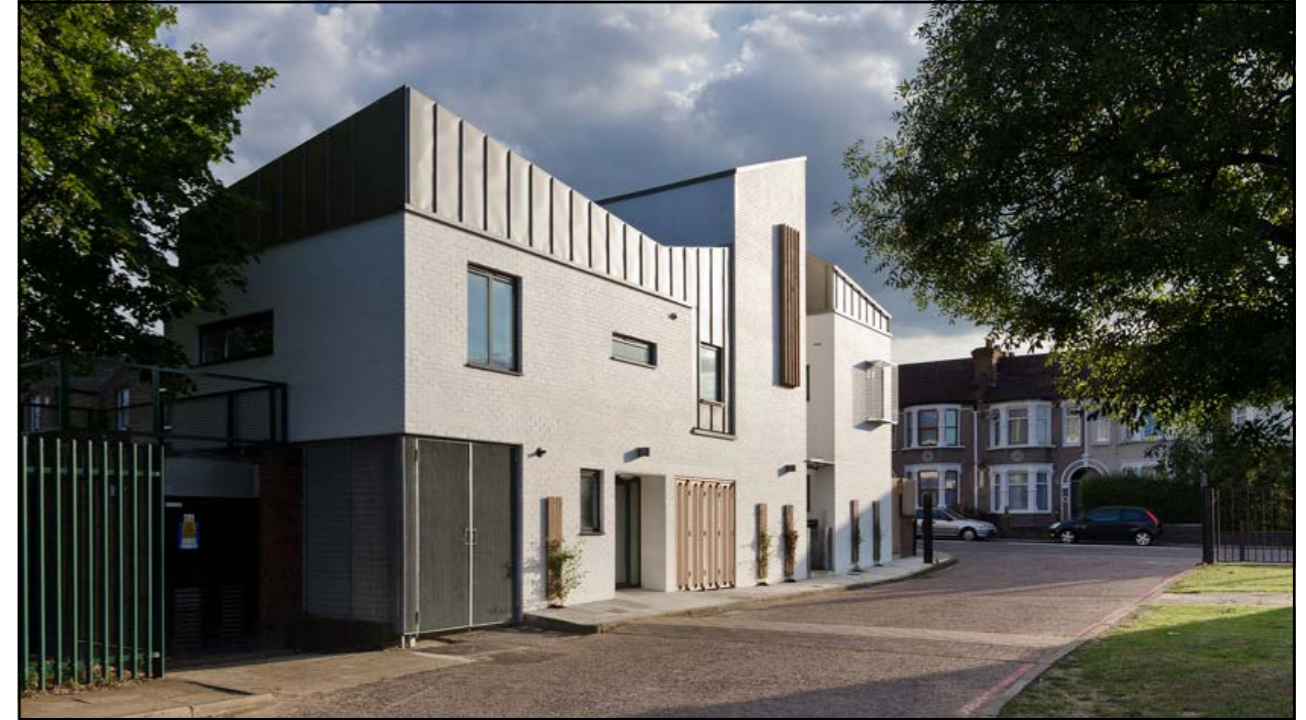
Fig. 137: The small residential development on the corner of two streets in Crofton Park replaces a school keeper's cottage with three flats and a small house. (website: www.chancedesilva.com , photography: Tim Crocker)
