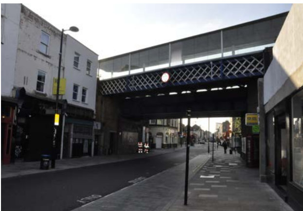
Fig. 22: Deptford Railway Station viaduct
