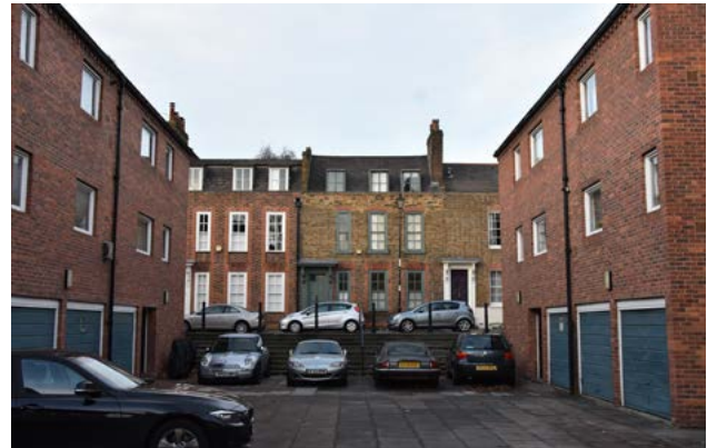
Fig. 82: Sunken ground level, Mary Ann Gardens
