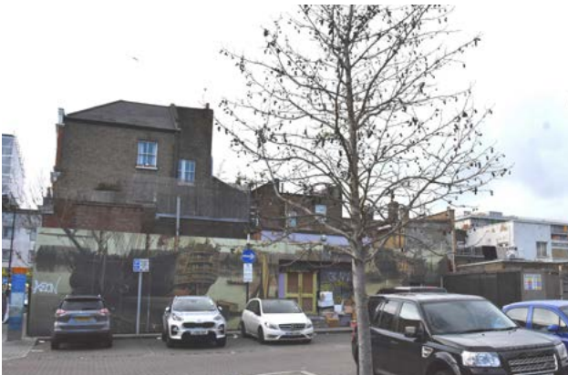
Fig. 37: Rear elevations on approach from Frankham Street
