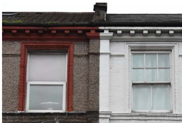
Fig. 177: Traditional timber sash windows (right) alongside replacement uPVC windows (left)
