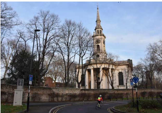
Fig. 91: Historic church wall
