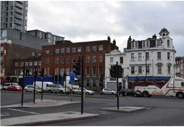
Fig. 150: Extension 4: Nos. 2- 16 Deptford Bridge
