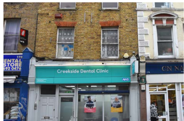
Fig. 173: Appropriately sized modern signage
