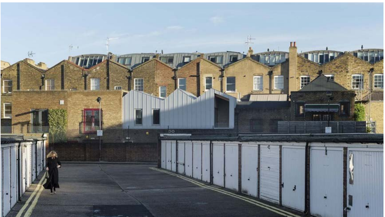
Fig. 181: In this example of rear plot development, the form of the roof responds to that of the historic houses on the front of the plots. The roof also expresses the plot boundaries, whilst the historic boundary wall is retained. The height of the development and the choice of materials means that the historic houses are still clearly understood to be the principal buildings on the plots, with their roofs and rear elevations visible from public areas.
