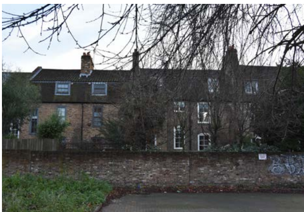
Fig. 85: Rear elevation of Albury Street seen from Creek Road
