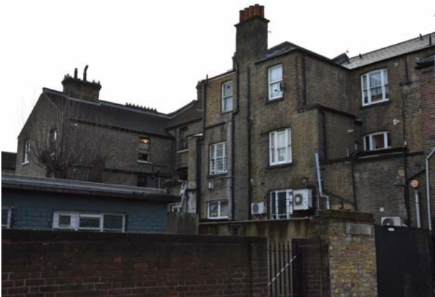
Fig. 77: Residential rear extensions to Deptford High Street
