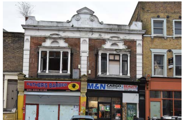
Fig. 49: At risk: Nos. 462-464 New Cross Road
