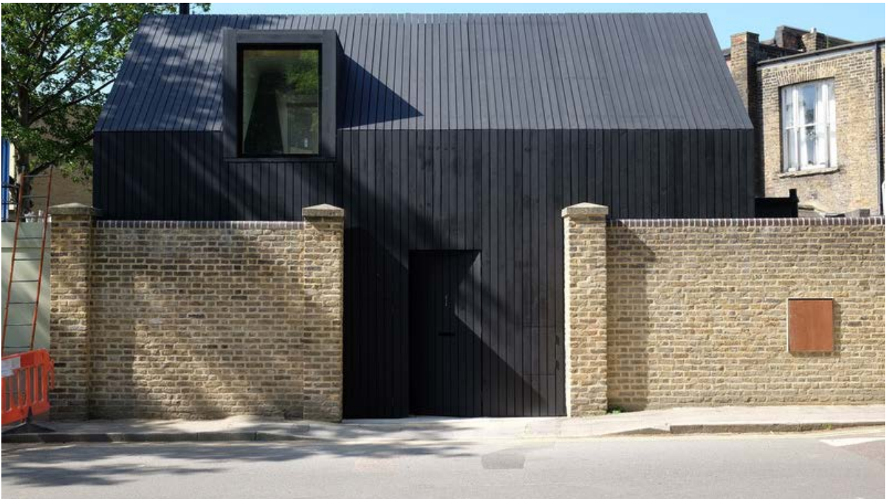
Fig. 180: This new house on Crossfield Street is a good example of best practice. The historic boundary wall is retained, and the building is lower than the frontage building and clearly of an ancillary form, allowing views of historic buildings on Deptford High Street behind. Although there are modern details, the design draws on local architectural traditions: the pitched roof is of a traditional form and the black-stained timber is inspired by buildings that were once common in Deptford, and materials used in the Royal Dockyard. The result is a development that creates an attractive environment for pedestrians and an appropriate setting for the Grade I listed St Paul's church.
