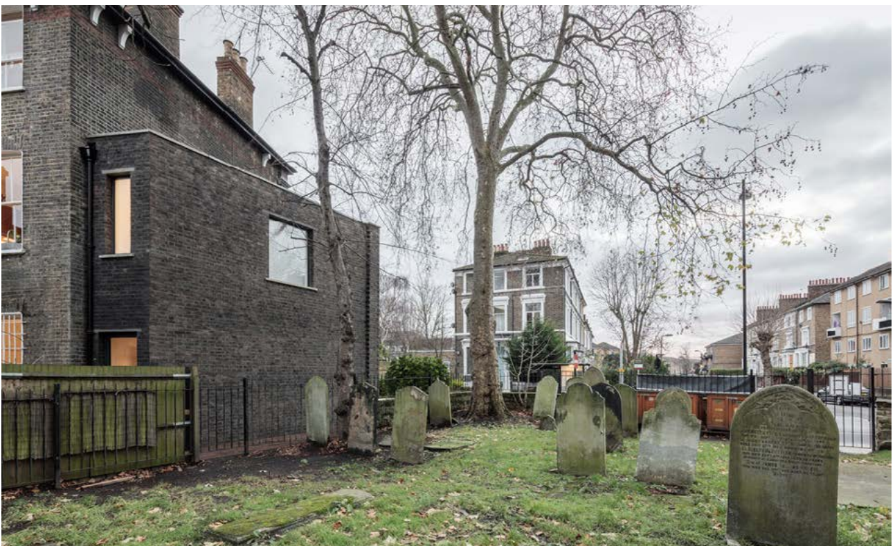
Fig. 179: Another example of good practice. This is clearly an ancillary extension, and has carefully matched brickwork and subtle detailing.
