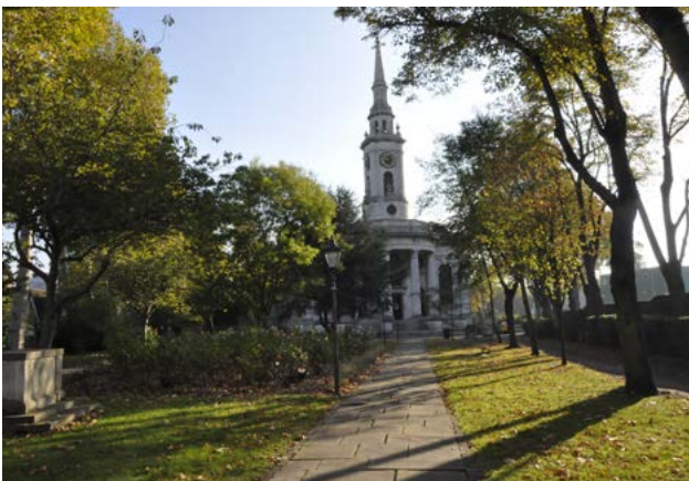
Fig. 14: St Paul's Church, view from west
