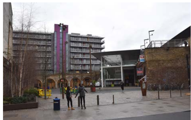
Fig. 64: Refurbished station area
