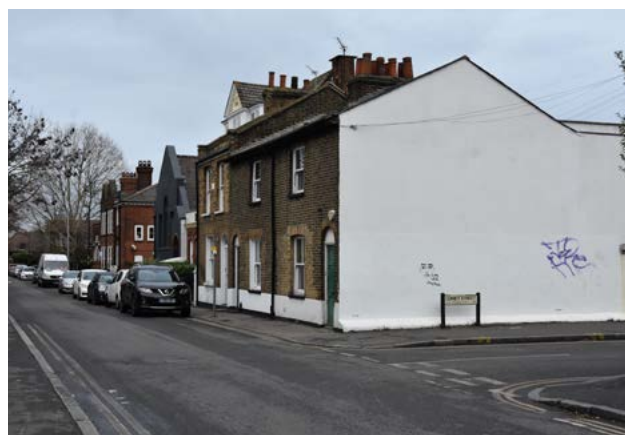
Fig. 72: Houses on Watson's Street
