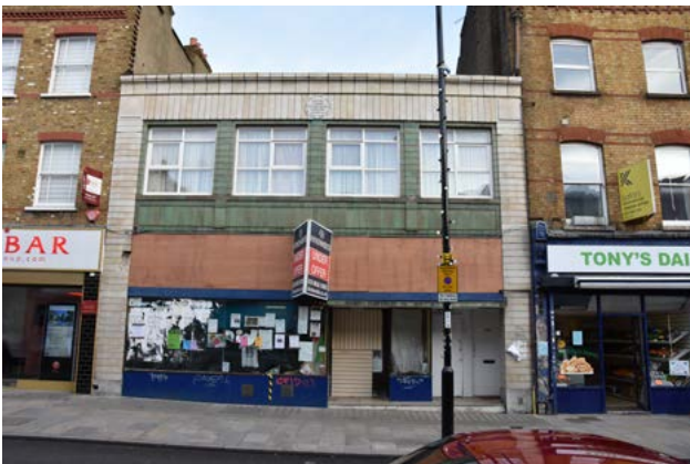
Fig. 48: At risk: No. 144A Deptford High Street
