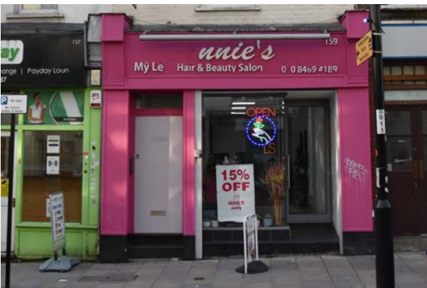
Fig. 169: Sensitively designed modern shopfront
