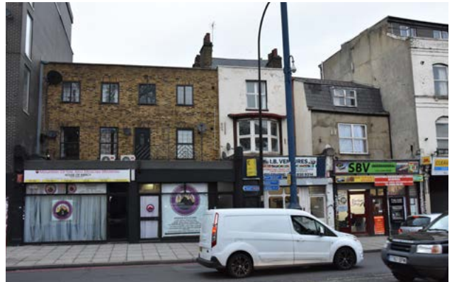
Fig. 153: Extension 5: Nos. 465-481 New Cross Road
