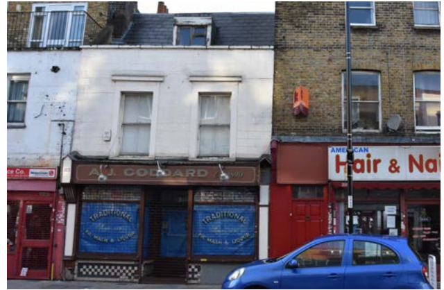
Fig. 47: At risk: pre-1800 building, unoccupied
