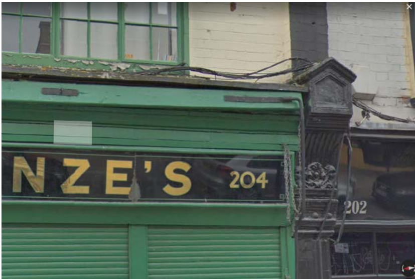
Fig. 165: Good quality historic shopfront details, 202 & 204 Deptford High Street
