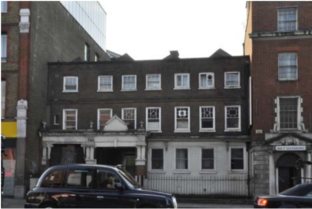
Fig. 46: At risk: Holland and Co. distillery (Grade II)
