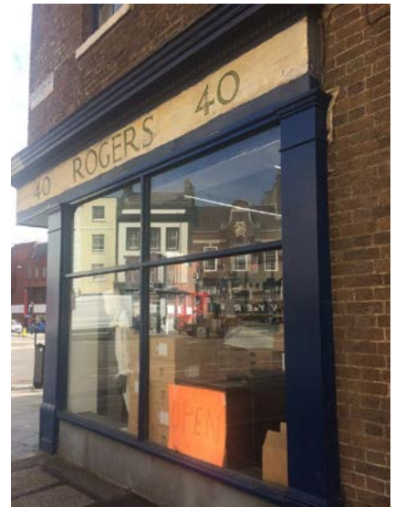
Fig. 166: High quality historic shopfront
