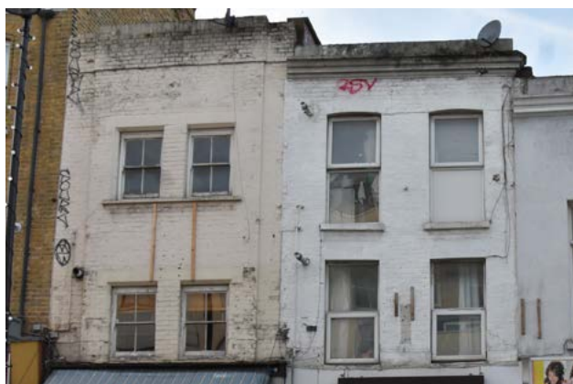
Fig. 176: Traditional timber sash windows (left) alongside replacement uPVC windows (right)
