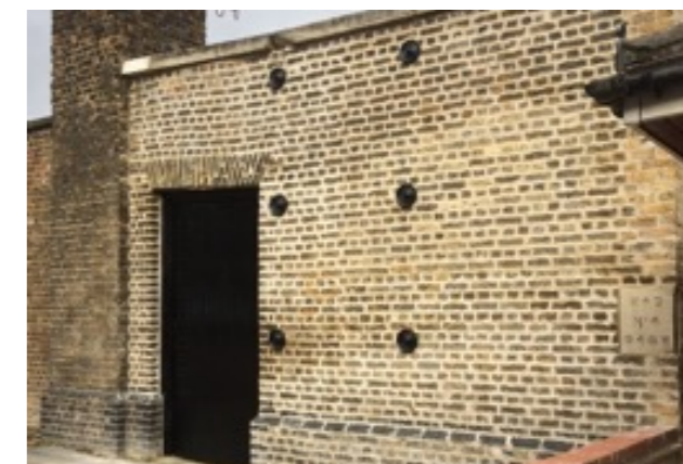
Photo 10: After the Grove Street wall repair Source: LB Lewisham
