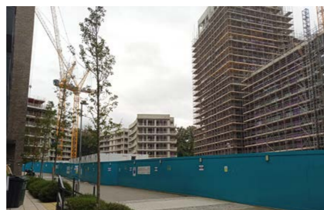
Photo 17: Construction at Heathside and Lethbridge
