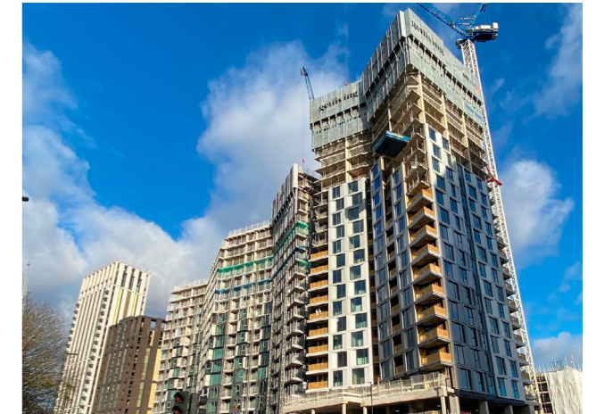
Photo 14: Phase 2 Lewisham Gateway Under Construction Source: LB Lewisham
