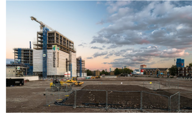
Photo 12: Timberyard Under Construction Source: LB Lewisham
