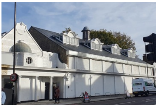
Photo 10: Works done at 233 - 241 Lewisham High Street (formerly Riley’s Snooker Hall) Source: LB Lewisham
