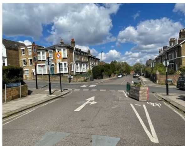
This photo shows the signage on Pascoe Road, including a 'No Left Turn' sign and arrows on the road that indicate motorists can proceed straight ahead or turn right.
