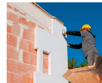
External wall insulation Grant & 100% free internal wall insulation
